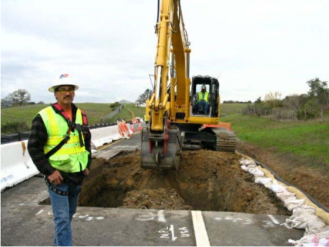
Figure 1 – Manhole #5 excavation along Cañada Road, Segment 1, February 14, 2005
