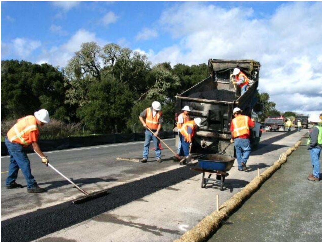
Figure 4 – Trench being paved between Manhole #7 and #8, Segment 1, February 18, 2005
