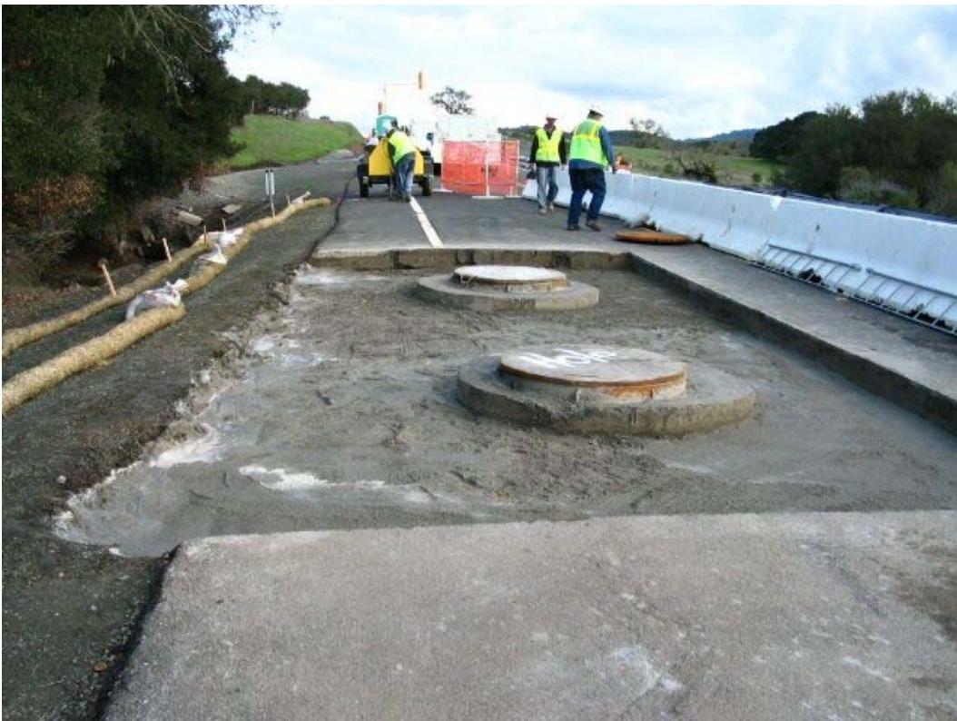
Figure 2 – Manhole #6 cement slurry poured and rings set, Segment 1, February 16, 2005
