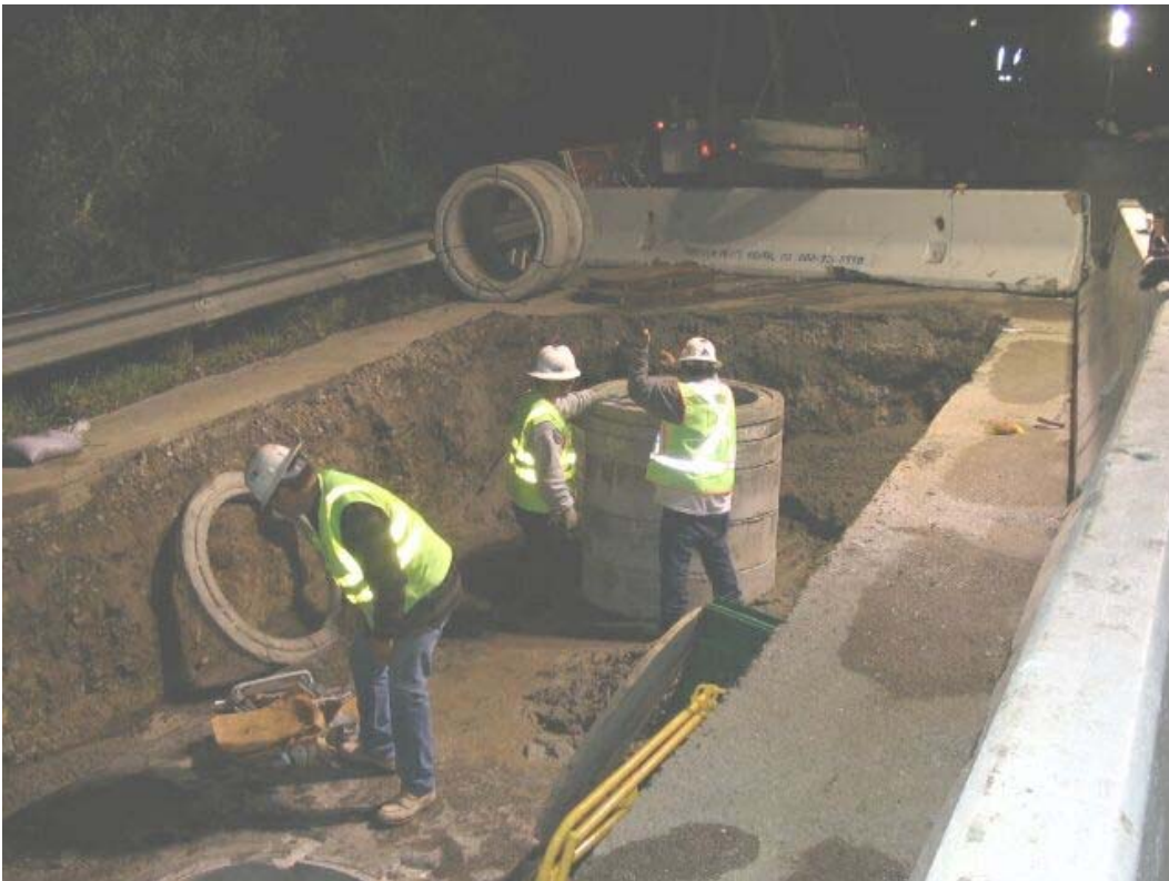
Figure 2 – Setting manhole rings at Manhole #20 in the Caltrans ROW, Segment 1, March 2, 2005
