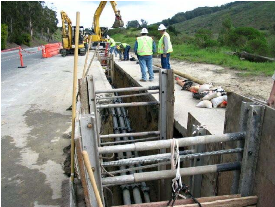
Figure 5 – Crews installing conduit in trench east of Manhole #68, Segment 5, March 3, 2005
