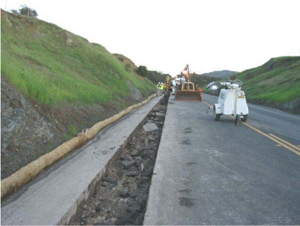
Figure 1 – Trenching along Cañada Road, Segment 1, February 28, 2005
