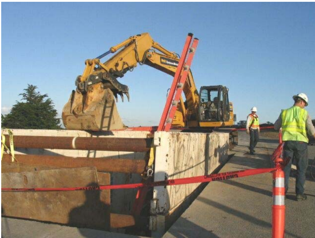
Figure 4 – Shoring Manhole #70 on Guadalupe Canyon Parkway, Segment 5, February 28, 2005
