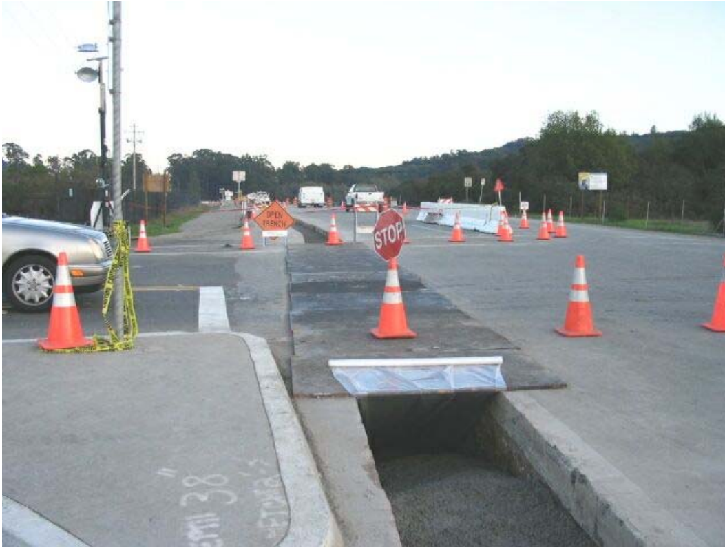
Figure 1 – Trench at Cañada Road and Edgewood Drive intersection, Segment 1, March 9, 2005
