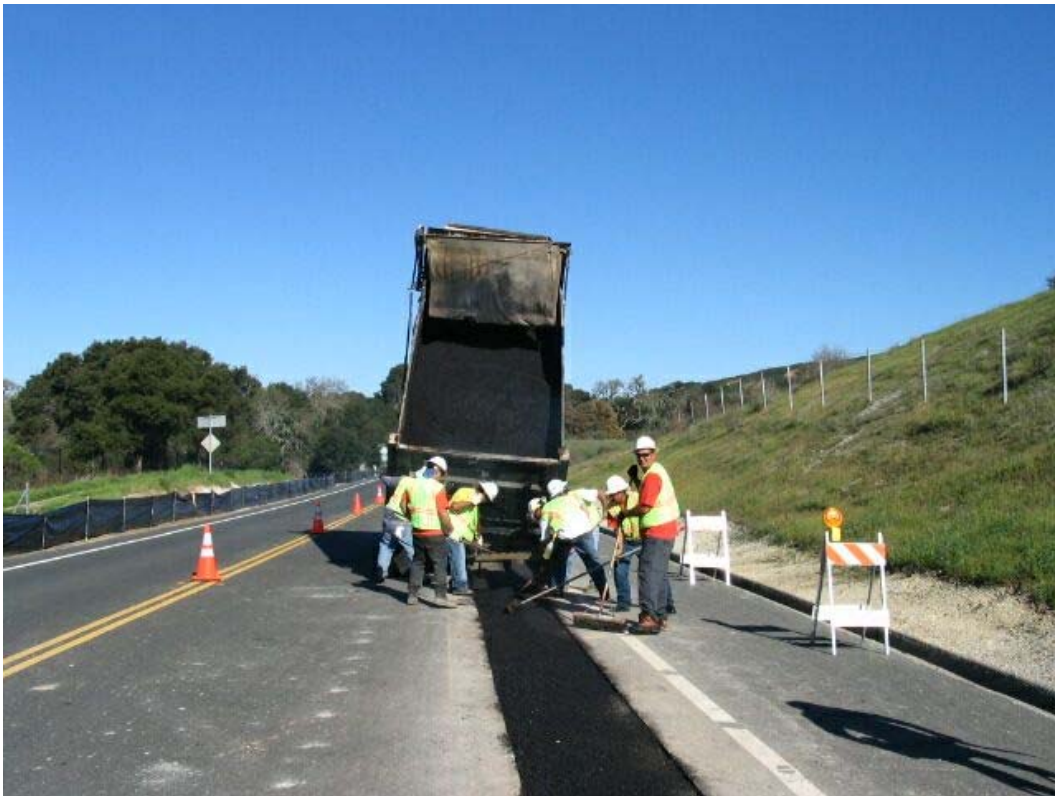
Figure 3 – Crews paving north of Edgewood Drive on Cañada Road, Segment 1, March 11, 2005
