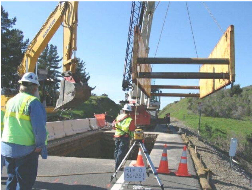
Figure 2 – Installing shoring at Manhole #10 along Cañada Road, Segment 1, March 7, 2005
