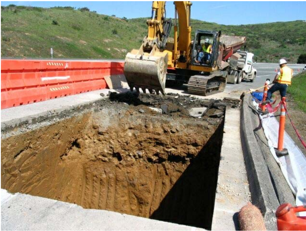
Figure 5 – Crews excavating Manhole #71 vault pit, Segment 5, March 7, 2005
