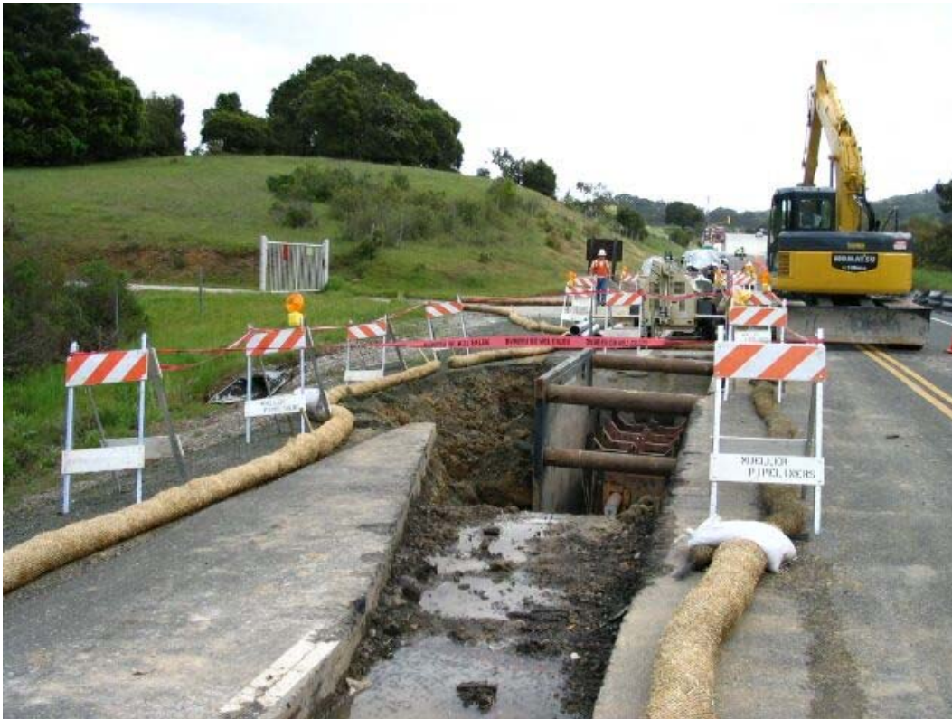
Figure 1 – Stub-out areas at Manhole #4 on Cañada Road, Segment 1, March 29, 2005.
