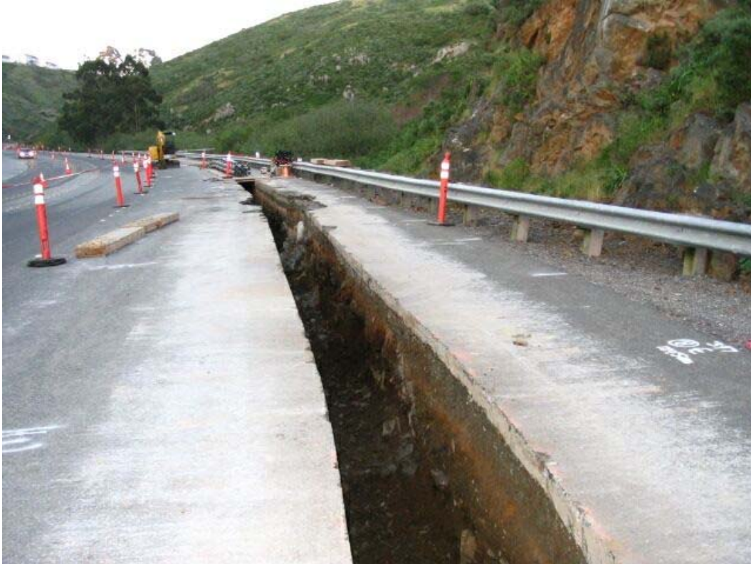
Figure 5 – Trench excavated east of Manhole #66 on Guadalupe Canyon Parkway, Segment 5, March 30, 2005.
