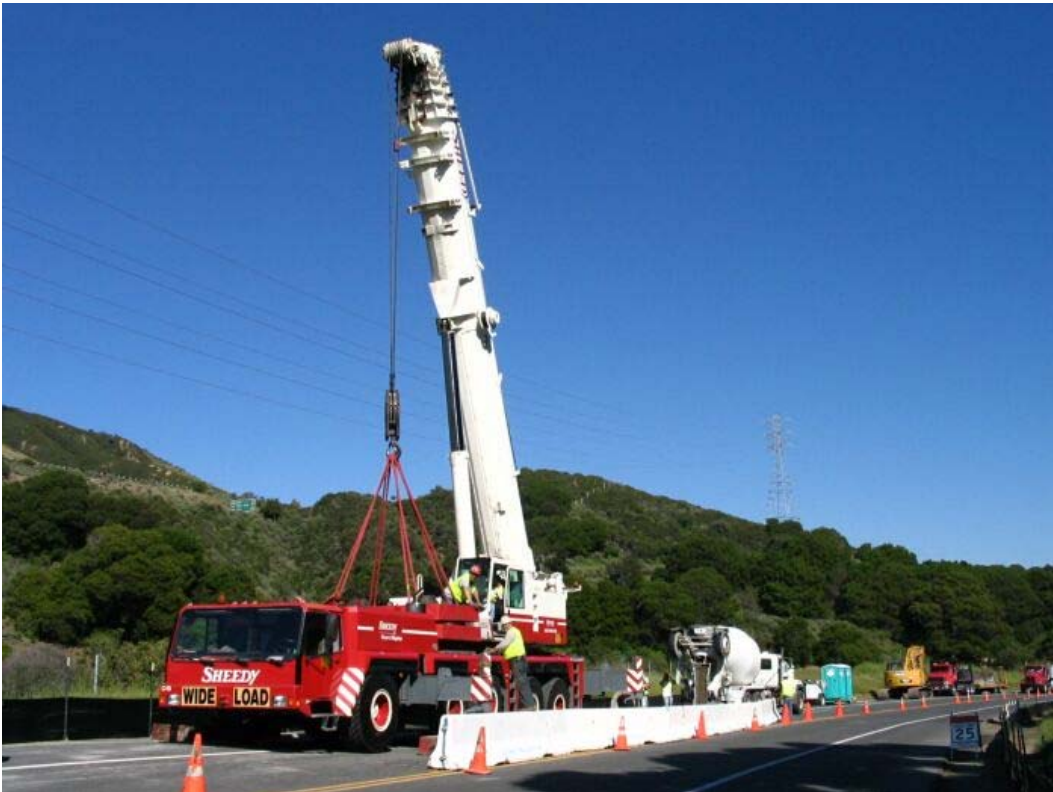
Figure 2 – Crane setting vault at Manhole #13 on Cañada Road, Segment 1, April 5, 2005.
