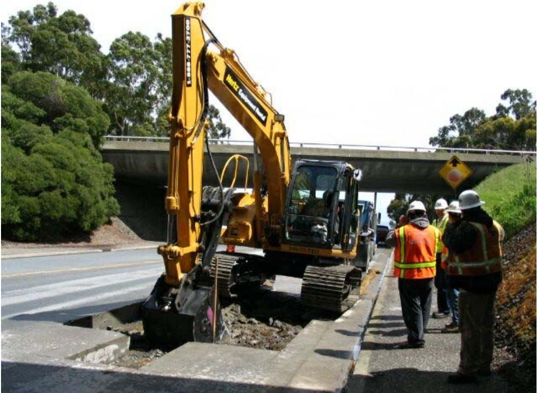
Figure 3 – Crews excavating asphalt for Manhole #37 on Trousdale, Segment 2, April 7, 2005.
