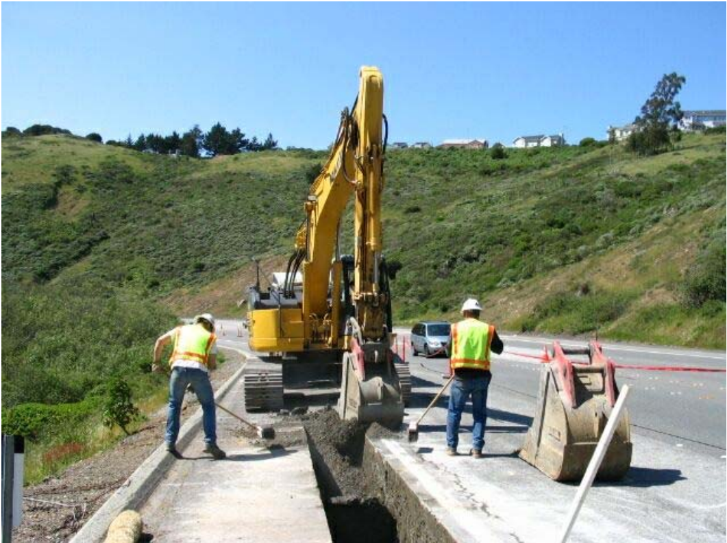
Figure 4 – Crews excavating east of Manhole #67 on Guadalupe Canyon Parkway, Segment 5, April 4, 2005.
