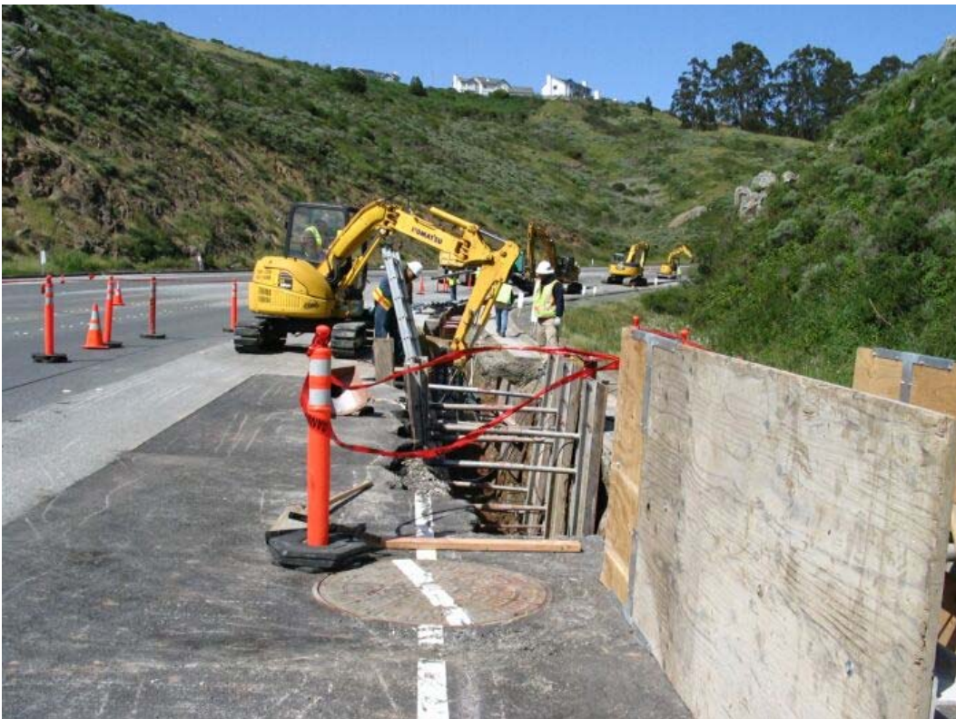
Figure 4 – Crews excavating east of Manhole #67 on Guadalupe Canyon Parkway, Segment 5, April 12, 2005.
