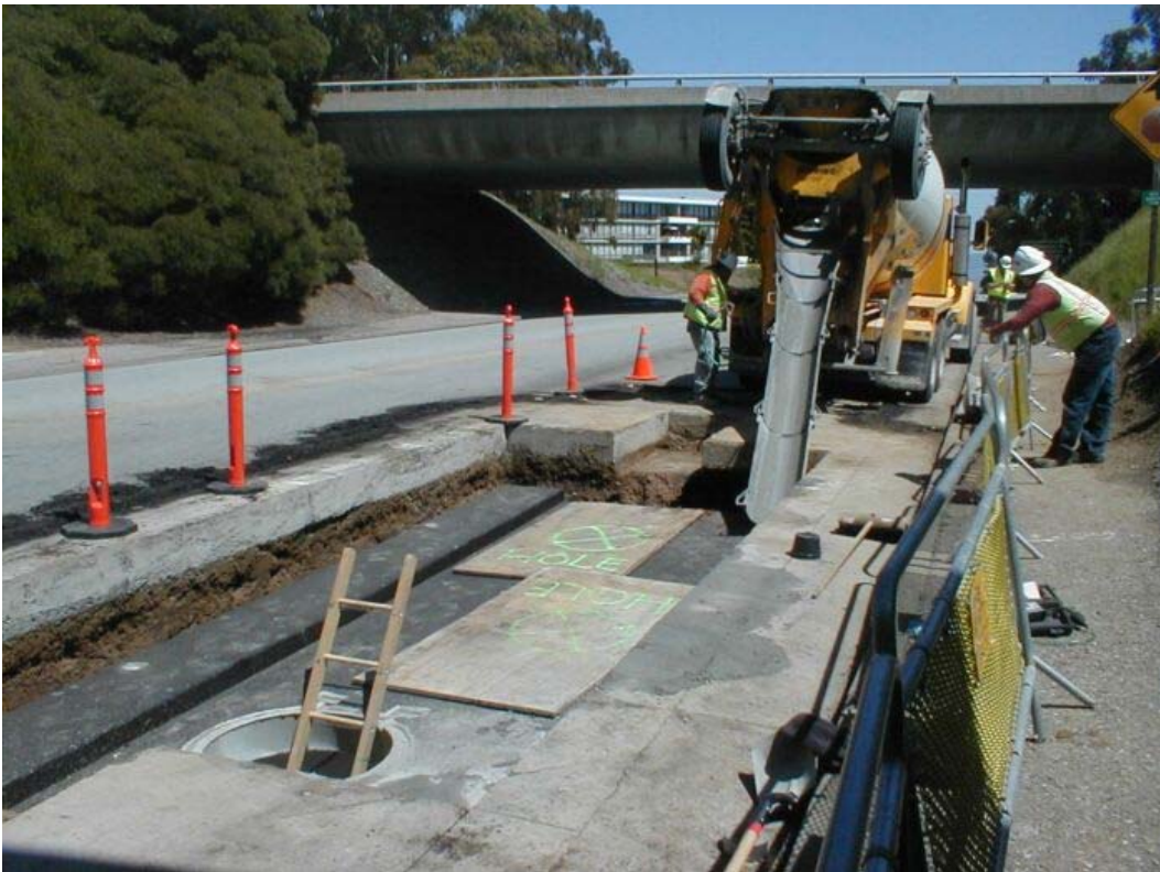
Figure 3 – Crews pouring cement slurry at Manhole #37 on Trousdale, Segment 2, April 14, 2005.
