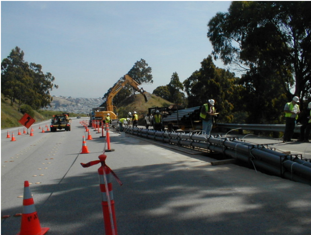
Figure 4 – Trenching activities east of Manhole #72 on Guadalupe Canyon Parkway, Segment 5, April 21, 2005
