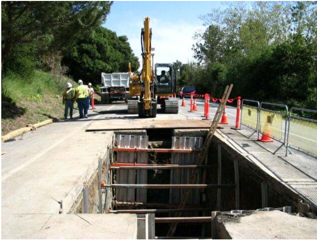
Figure 3 – Crews installing shoring at Manhole #35 on Skyline Boulevard, Segment 2, April 21, 2005.
