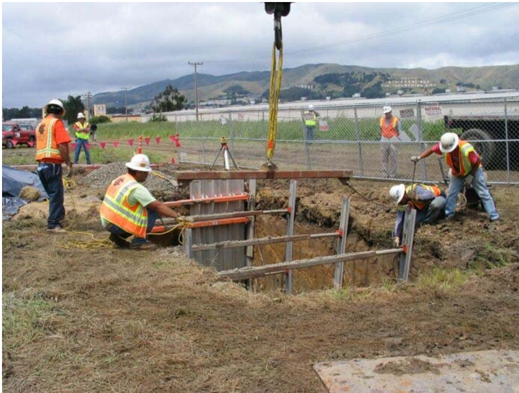
Figure 3 – Crews working at Manhole #49 in the BART right-of-way, Segment 4, May 5, 2005.
