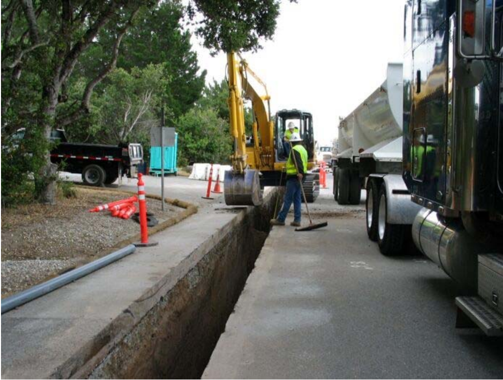
Figure 1 – Crews trenching between Manhole #8 and Manhole #9, Segment 1, May 17, 2005
