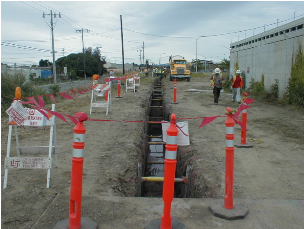
Figure 3 – Trenching area south of Manhole #48 in the BART right-of-way, Segment 4, May 18, 2005
