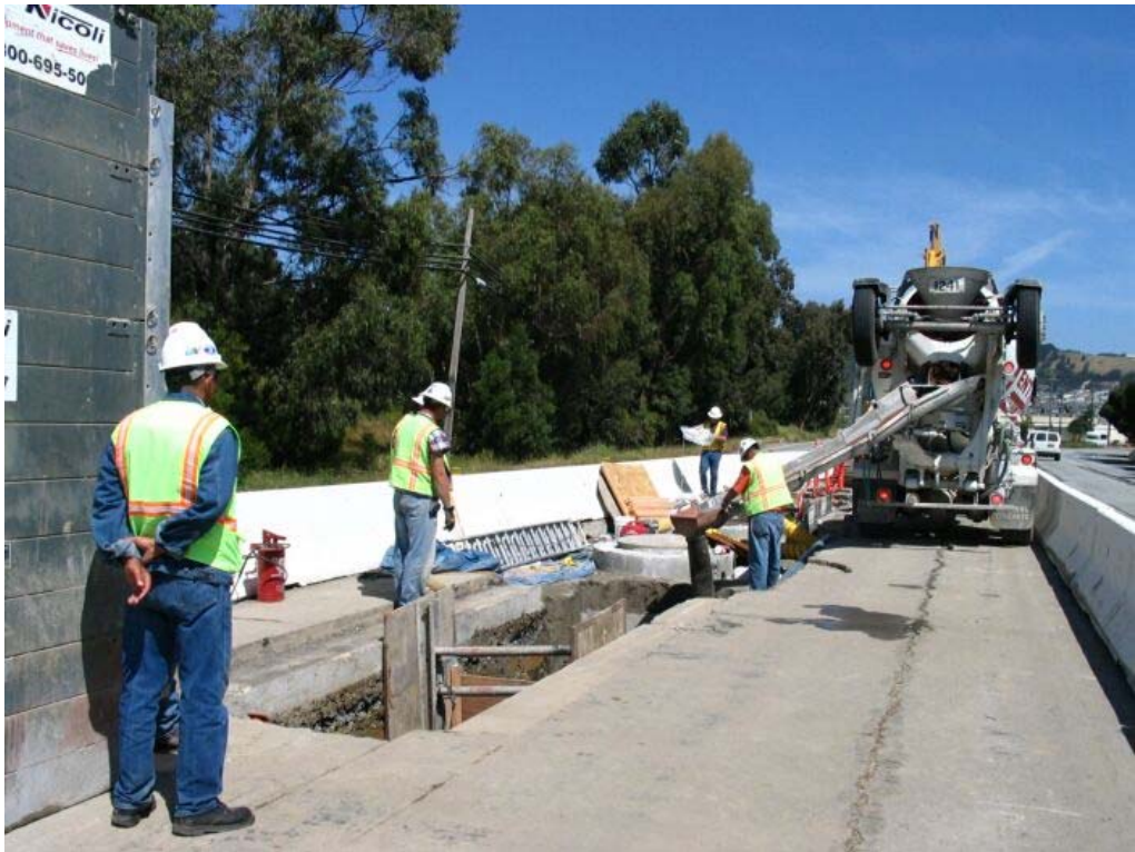
Figure 4 – Crews working at Manhole #78 on Bayshore Boulevard, Segment 5, May 20, 2005
