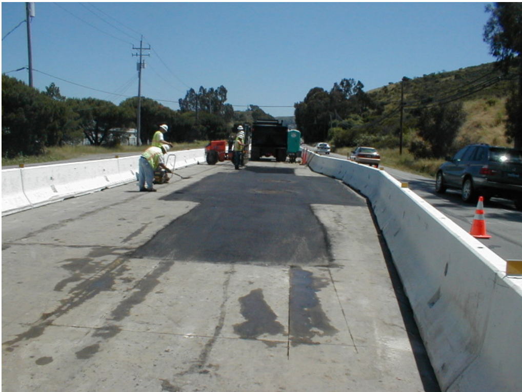
Figure 4 – Crews finishing paving at Manhole #78 on Bayshore Boulevard, Segment 5, May 25, 2005
