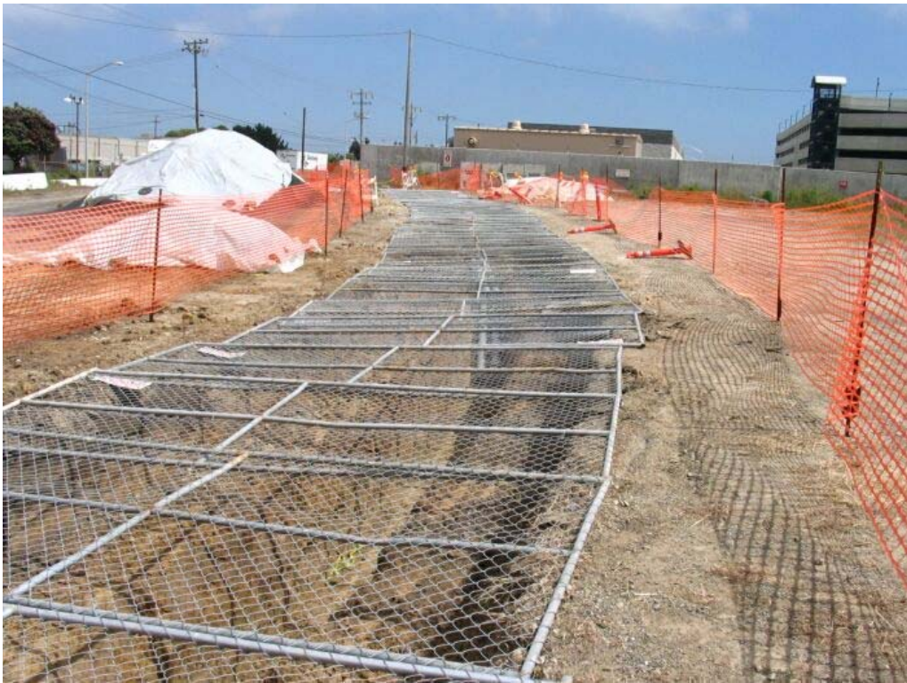
Figure 3 – Trenching area north of Manhole #48 in the BART right-of-way, Segment 4, May 27, 2005
