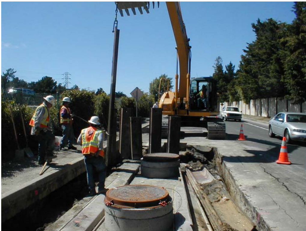
Figure 2 – Crews removing shoring at Manhole #30 on Skyline Boulevard, Segment 2 Underground, June 7, 2005
