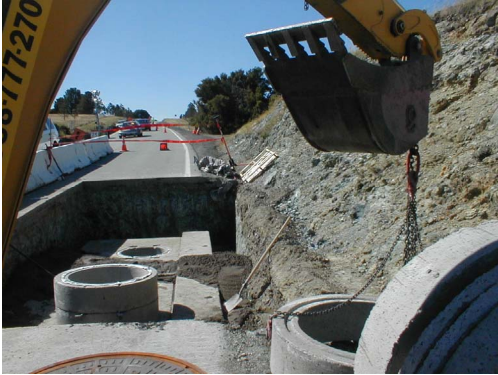
Figure 1 – Ring placement at Manhole #26, Segment 1, June 7, 2005
