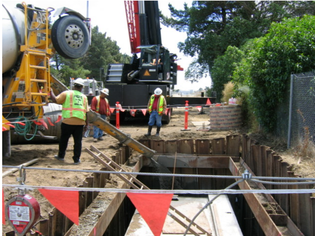
Figure 4 – Shoring and vault placement at Manhole #53, in Segment 4, June 9, 2005.
