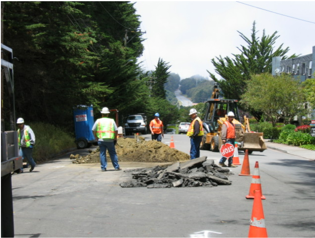
Figure 3 – Crews potholing near Manhole #39 Segment 3, June 9, 2005
