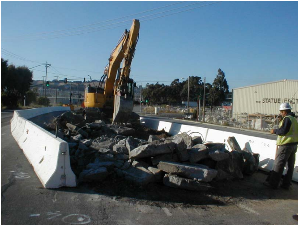
Figure 5- Segment 5 along Bayshore Boulevard in the City of Brisbane, June 6, 2005
