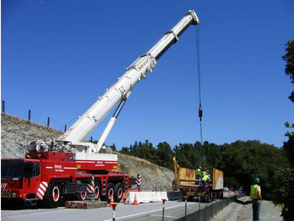
Figure 1 – Removing shoring at Manhole #24 with a large crane, Segment 1, June 14, 2005
