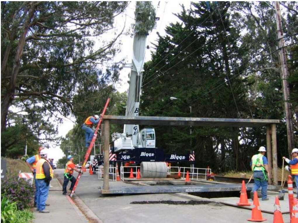
Figure 3 – Crews dismantling and removing shoring from Manhole #39, Segment 3, June 17, 2005
