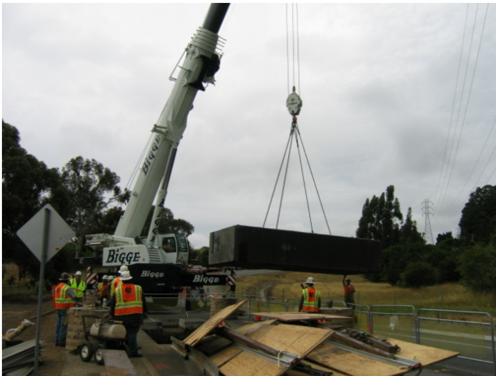
Figure 2 – Crews installing Manhole #28 on Skyline Boulevard, Segment 2 Underground, June 16, 2005
