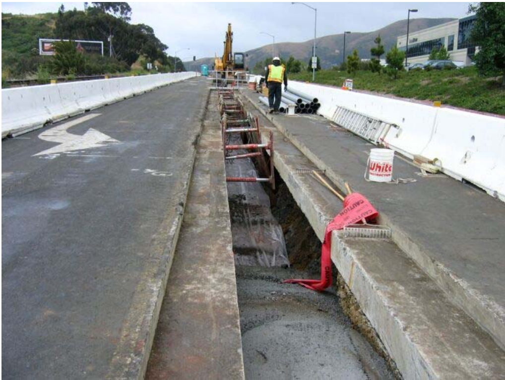
Figure 5- Trench along Bayshore Boulevard in the City of Brisbane, Segment 5, June 16, 2005
