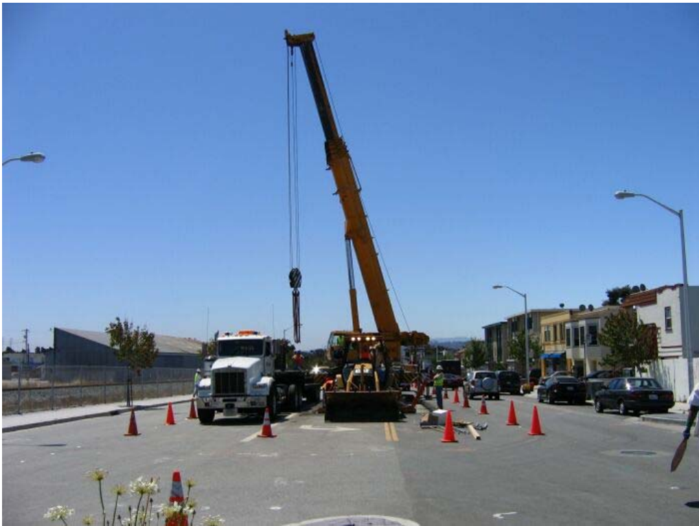
Figure 3 – Crews setting Manhole #46 on Huntington Avenue with large crane, Segment 3, July 1, 2005
