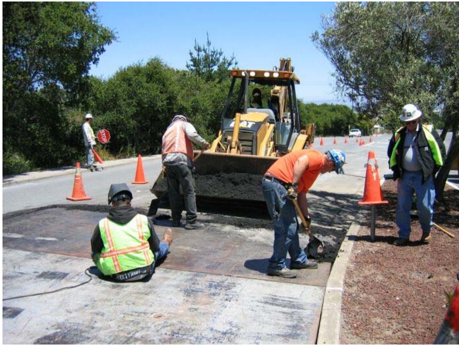
Figure 3 – Crews plating Manhole #40 on San Bruno Avenue, Segment 3, July 8, 2005
