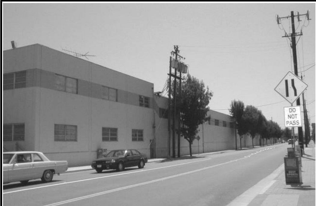
Photo B. View of West Face of Building from Across Hollis Street.
