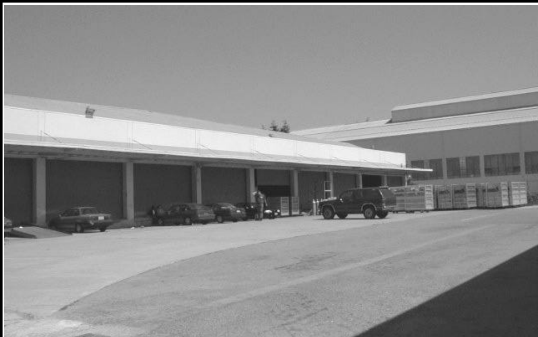
Photo C. On-Site View of South Face of Building.
