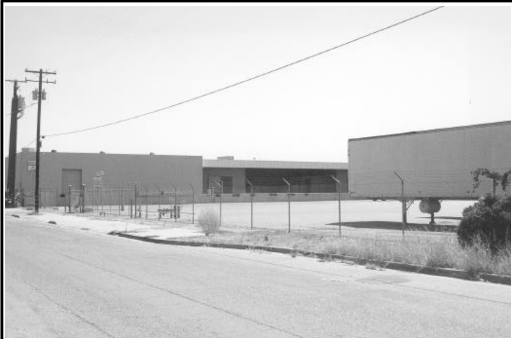
Photo A. Overall View of Site. Note that the site is fenced and there is light landscaping along W. Napa Avenue.
