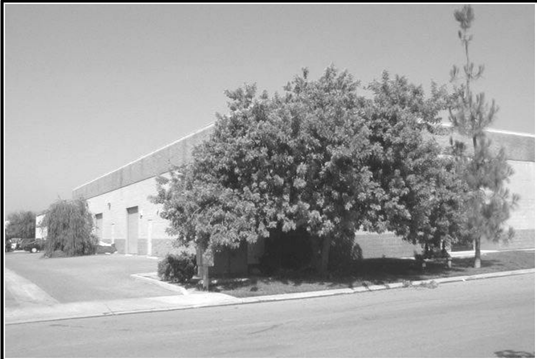
Photo C. South Face of Building.
