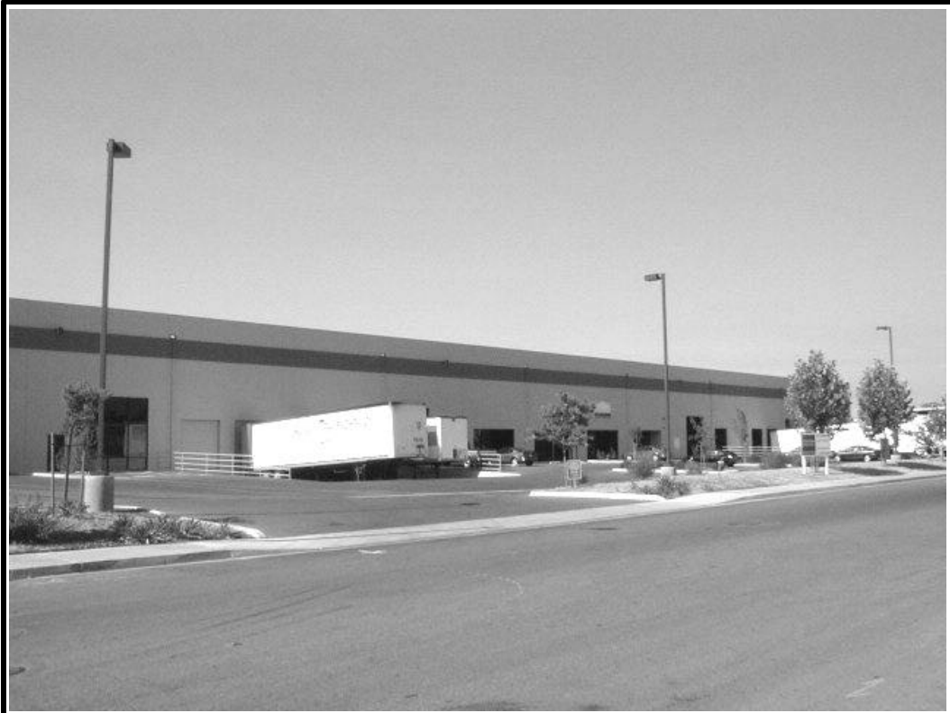
Photo C. View of North Face of Building Looking Southwest.
