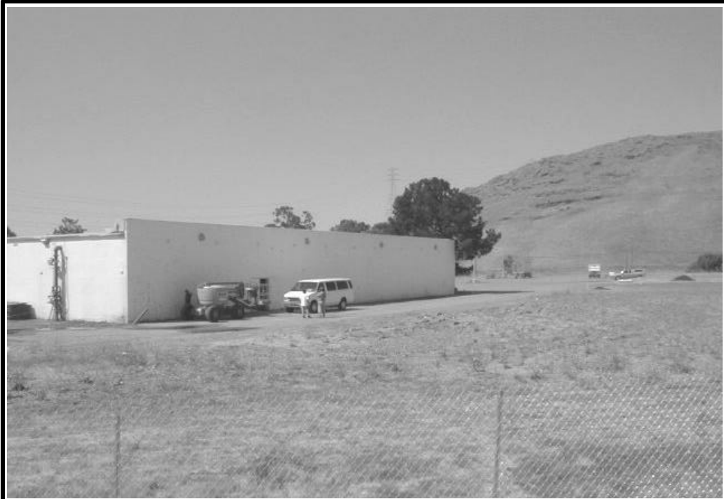
Photo E. North Face of Building, Proposed New Entrance Location
