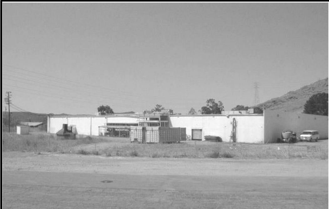
Photo B. View of East Face of Building.
