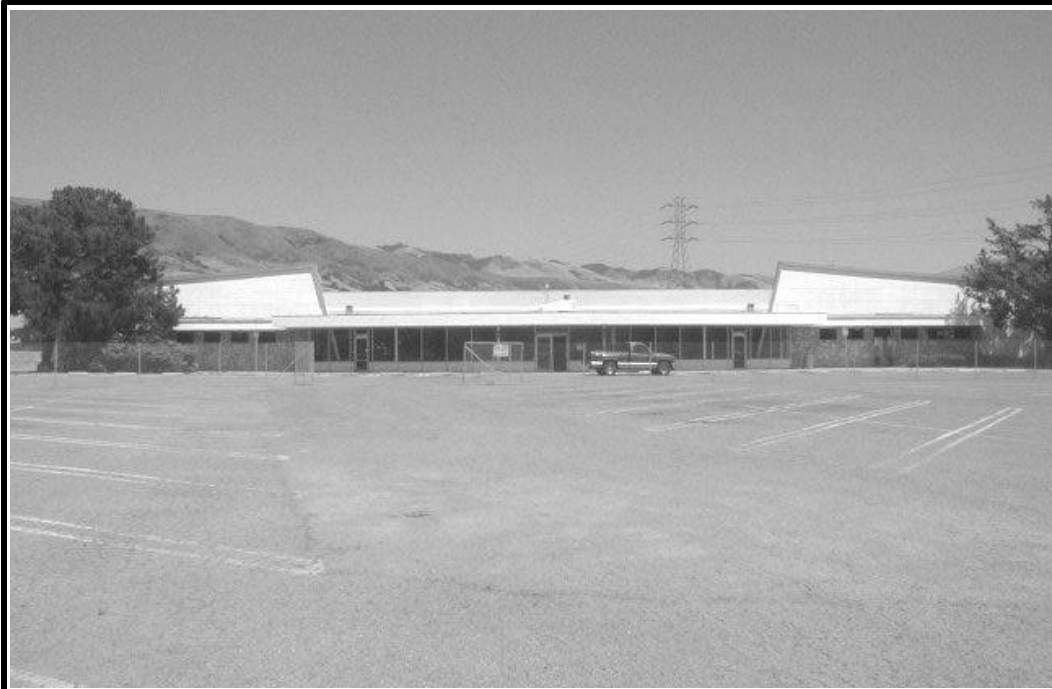
Photo A. View of West Face of Building.
