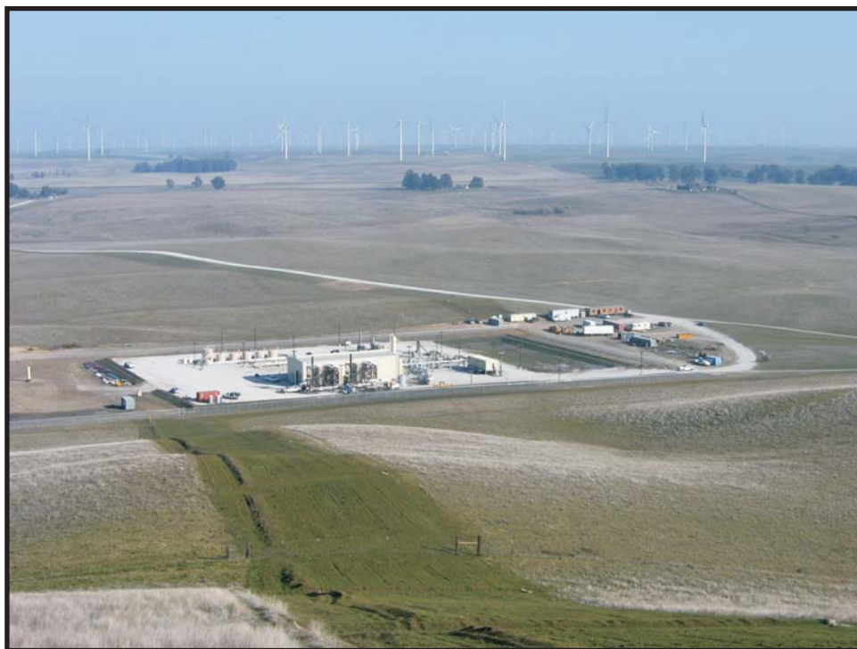
Kirby Hills Phase I Compressor Station Facility, January 23, 2007
