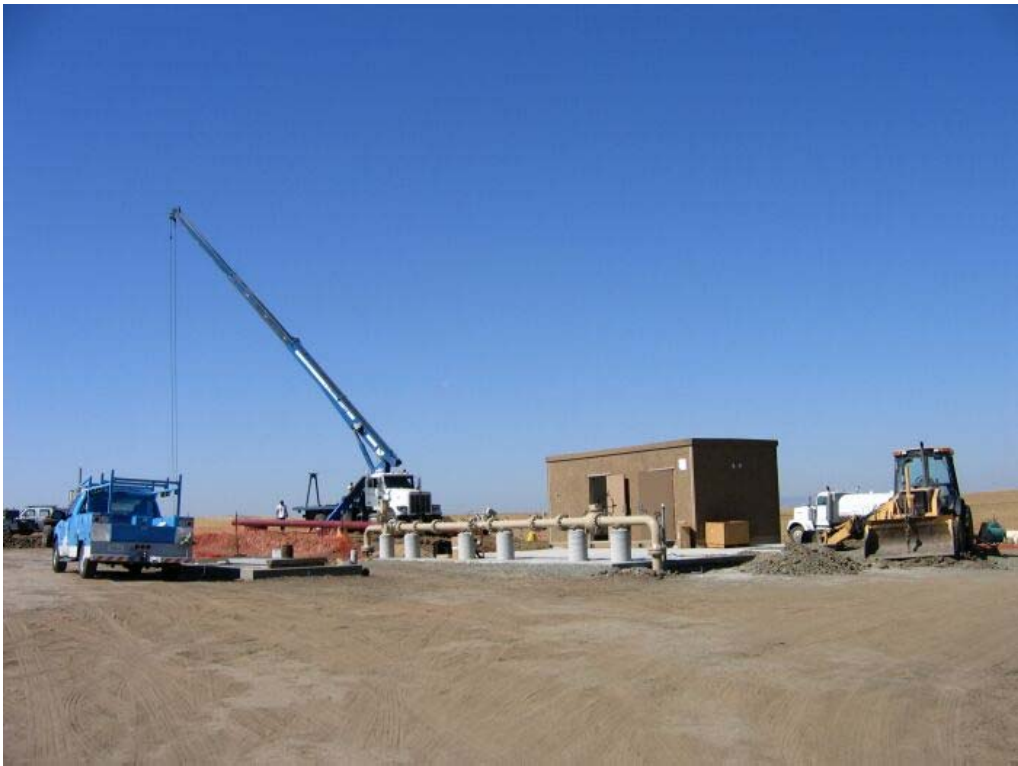
Figure 5 – Crews working on pipe installation at the Metering Station, October 12, 2006.
