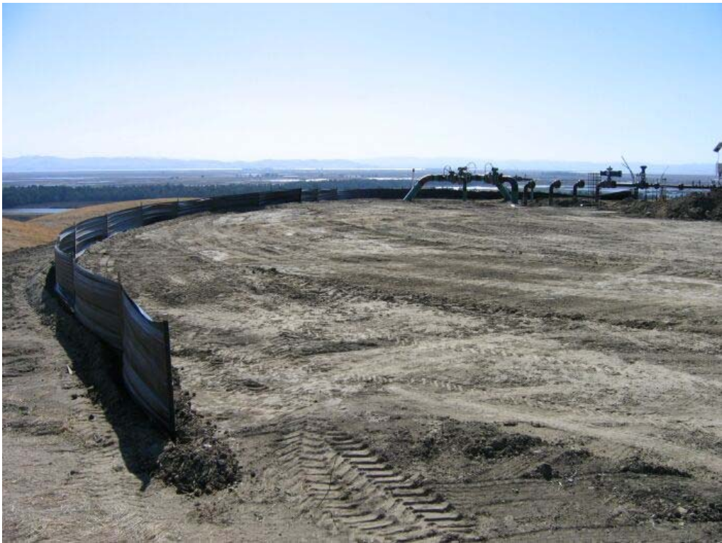
Figure 3 – Silt fence partially installed at well site S-10, October 10, 2006.
