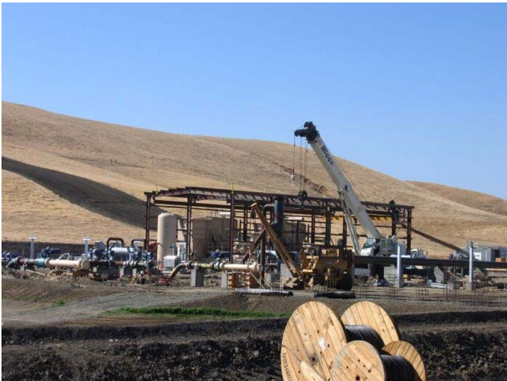
Figure 4 – Compressor building being erected at the Compressor Station, October 10, 2006.
