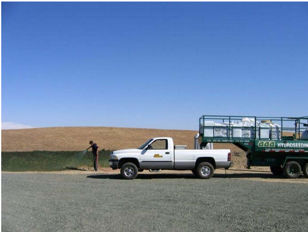
Figure 2 – Hydro-seeding at well site S-10, October 10, 2006.
