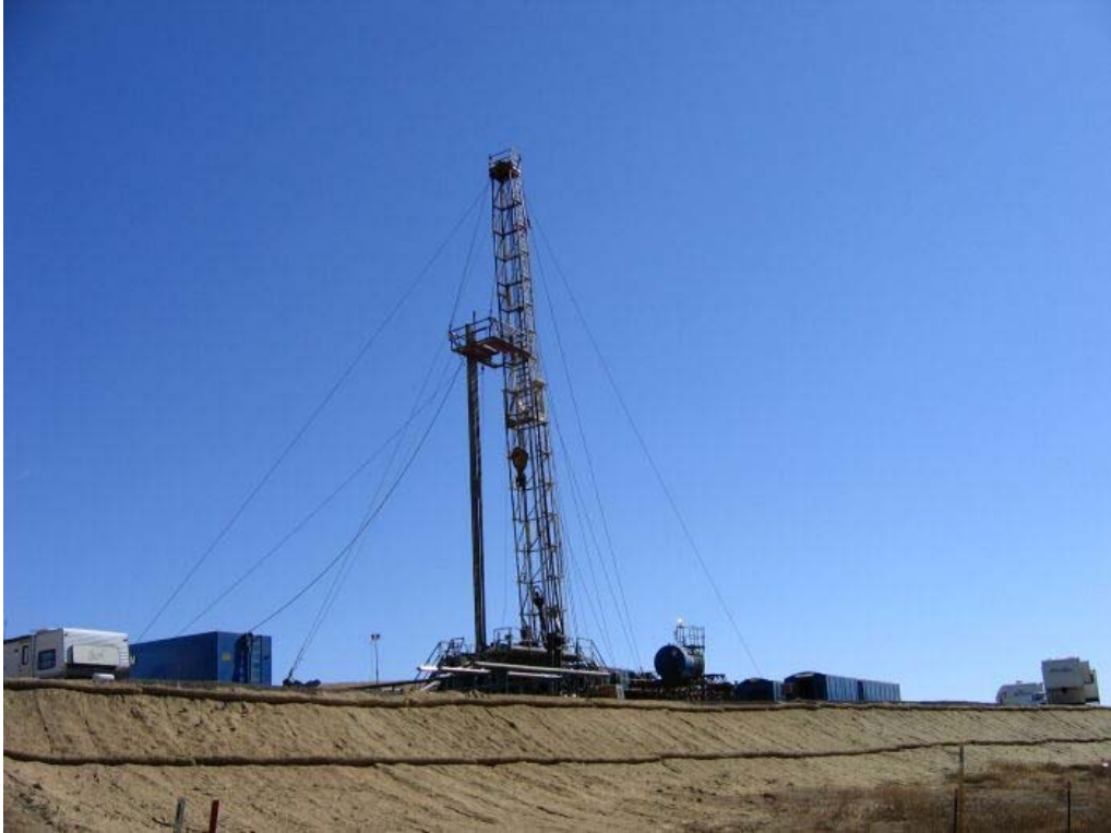
Figure 1 – Drilling rig set up at well site S-1, October 20, 2006.
