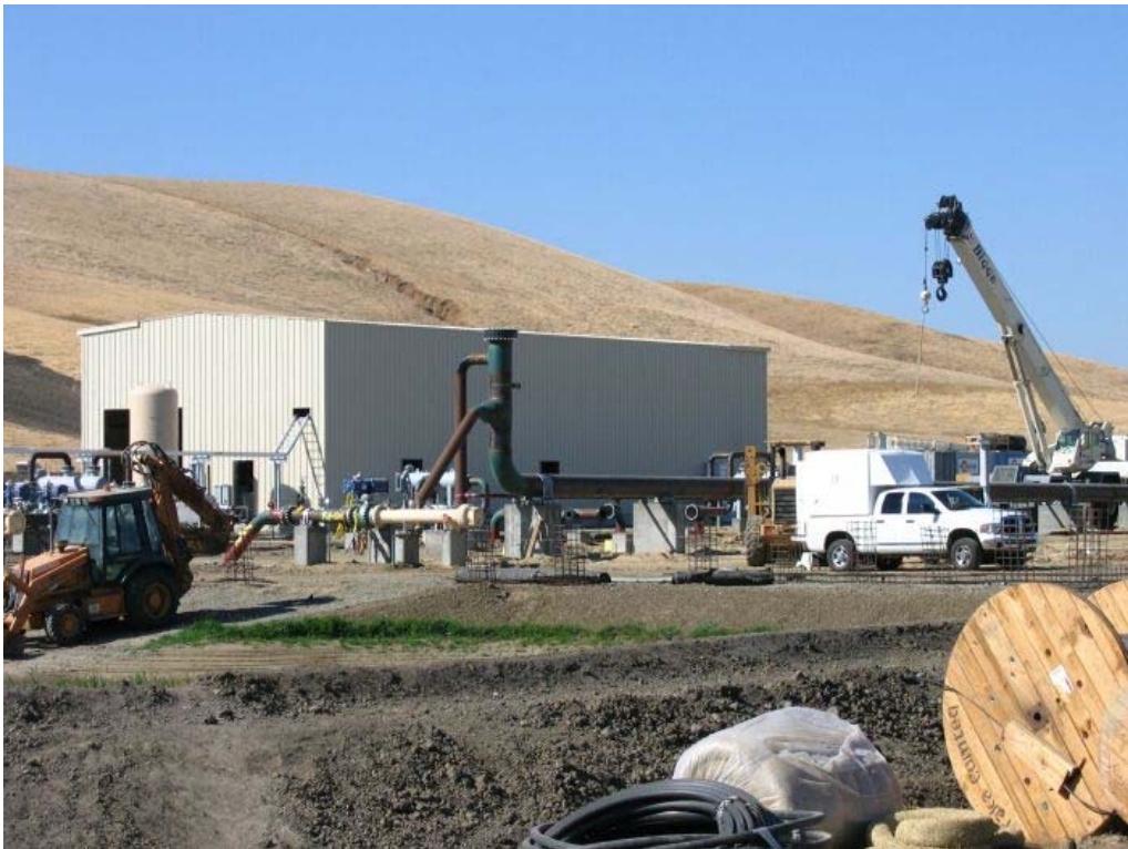
Figure 2 – Compressor building at Compressor Station, October 20, 2006.
