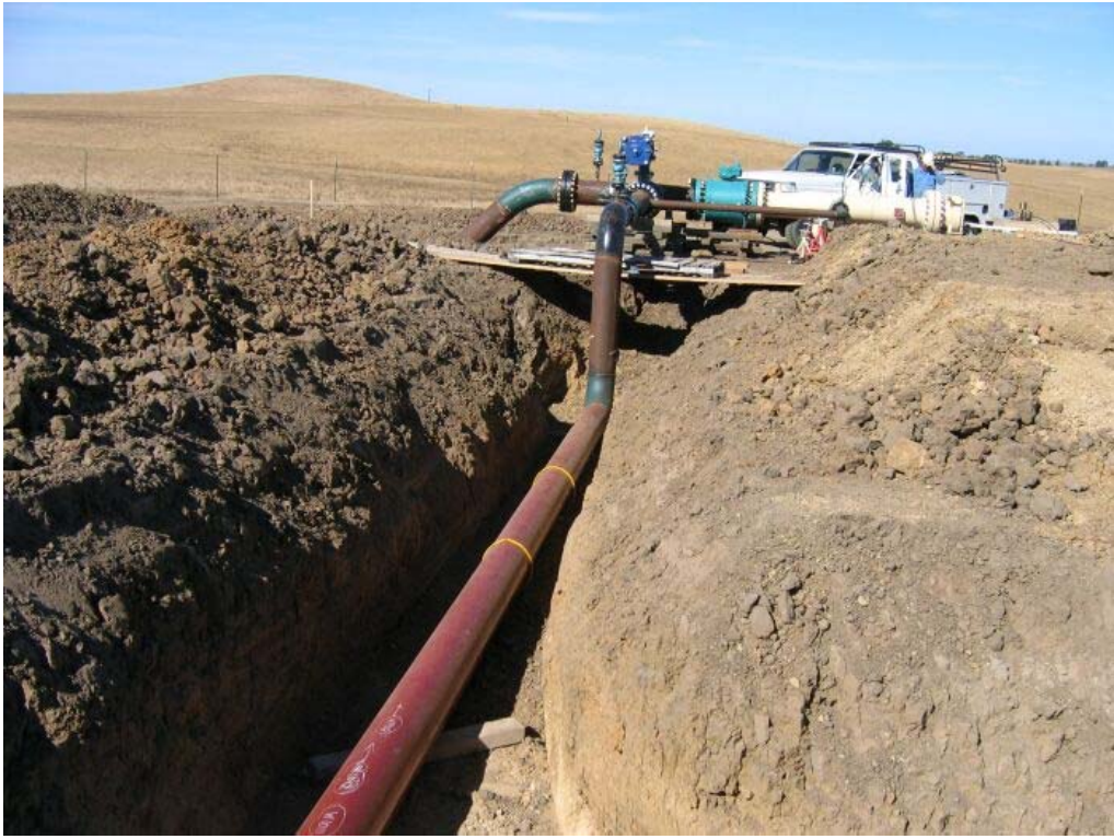
Figure 3 – Crews doing hydrostatic testing at the Metering Station, October 18, 2006.
