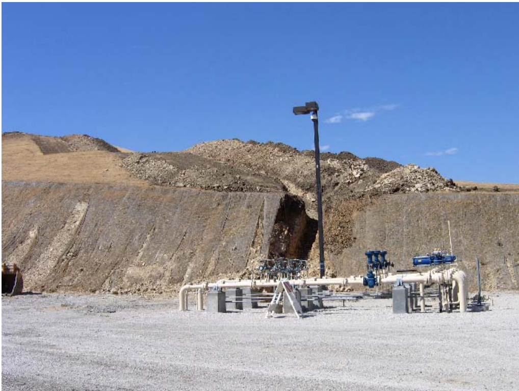
Figure 2 – Right-of-way and trench from Well Site S-2 to S-5. August 30, 2007.
