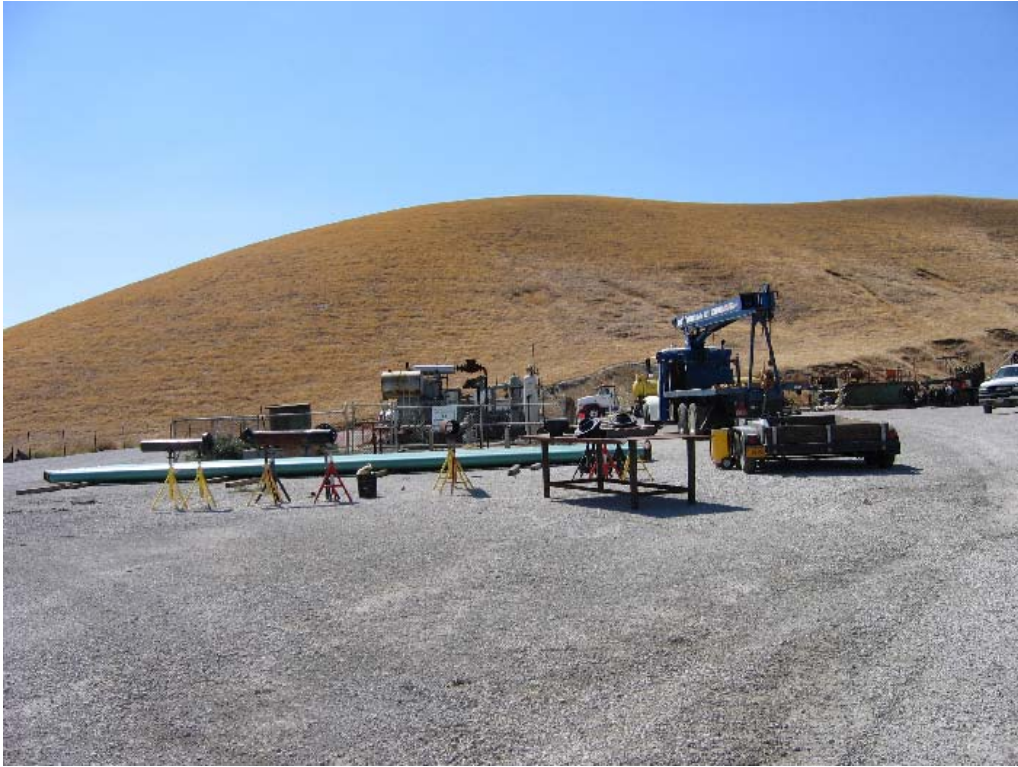
Figure 1 – Crews fabricating pipe at Well Site S-2. August 30, 2007.
