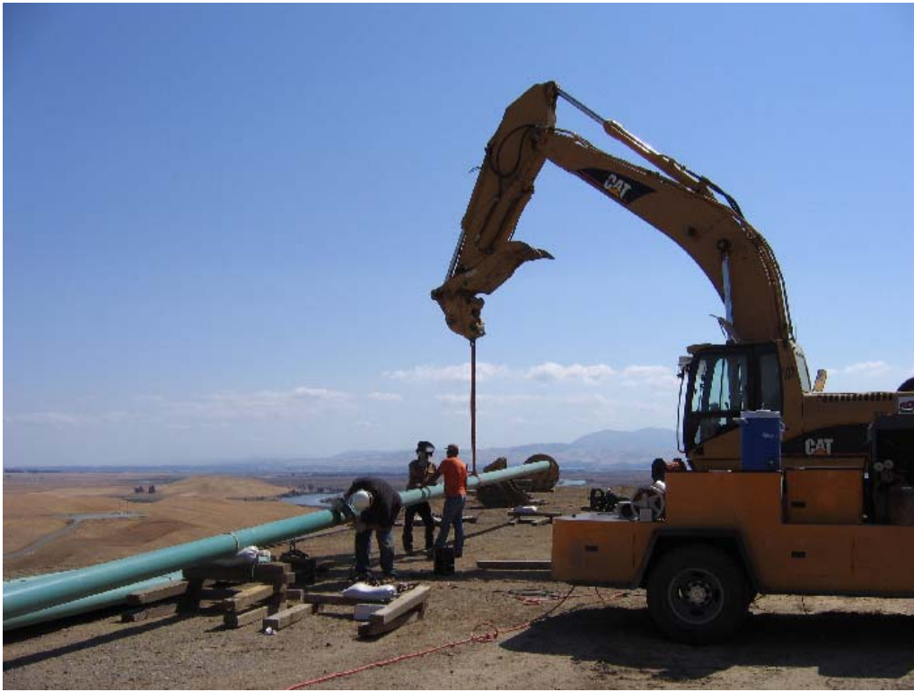
Figure 3 – Crews welding pipe at Well Site S-5. September 14, 2007.
