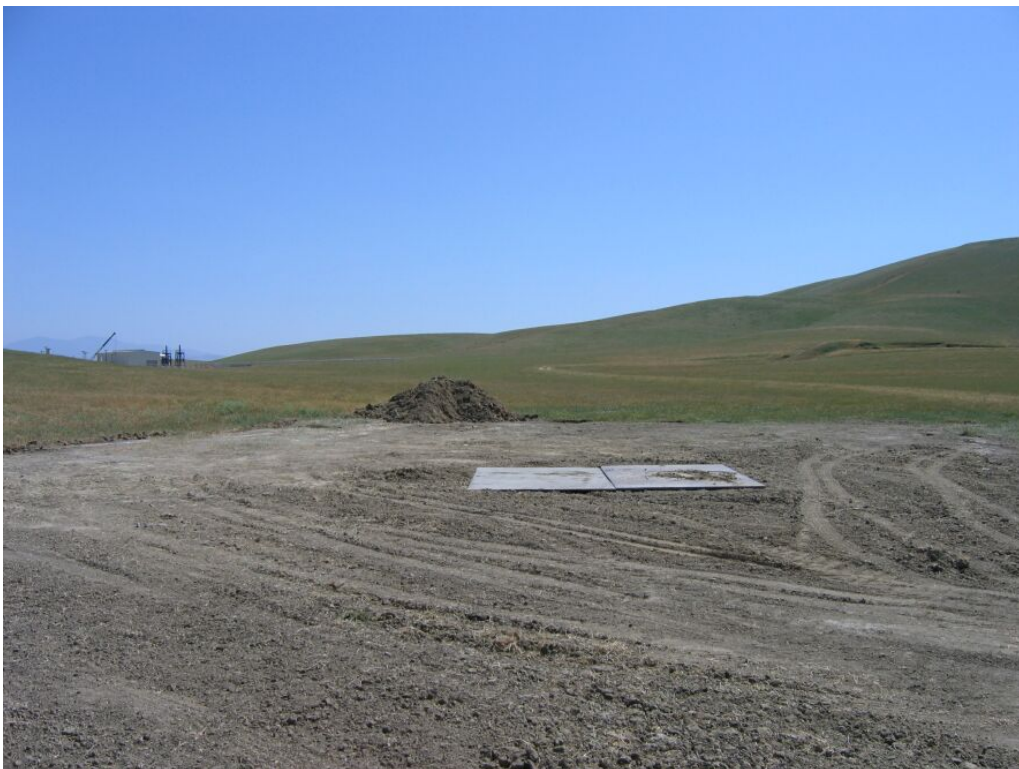
Figure 4 – Well L6 cleared and graded with trench plate coving hole, May 6, 2008.
