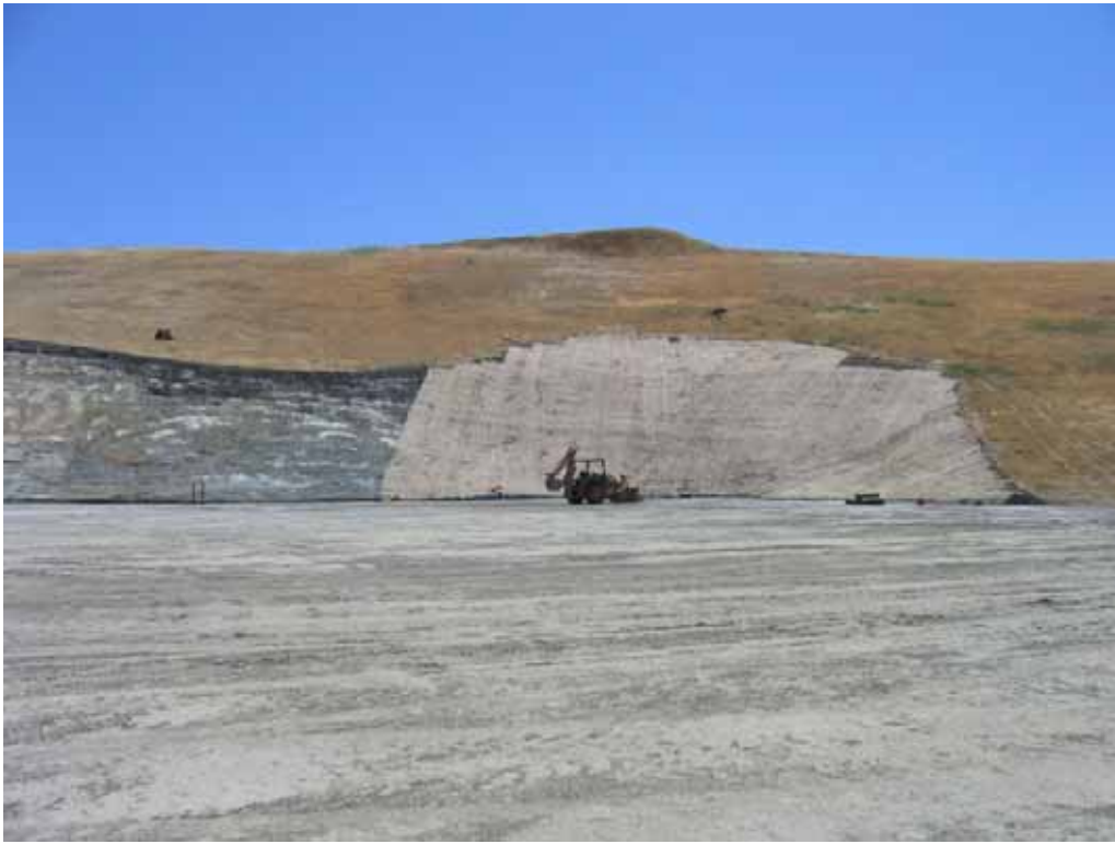
Figure 3 – Crew installing jute matting at WS-23, June 6, 2008.
