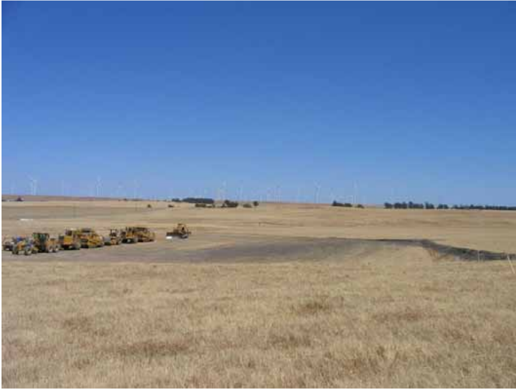
Figure 1 – Clearing and grading of Well Site 21, June 6, 2008.
