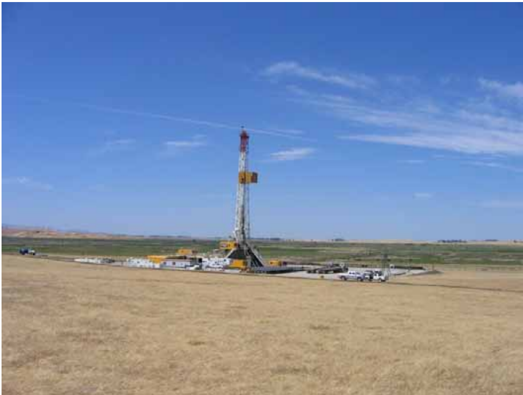
Figure 2 – Drill rig at WS-22, June 6, 2008.
