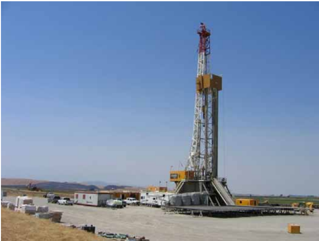
Figure 2 – Drill rig drilling at WS-22, June 13, 2008.
