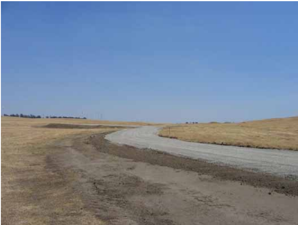
Figure 4 – Access road gravelled from WS-22 to WS-21, June 13, 2008.
