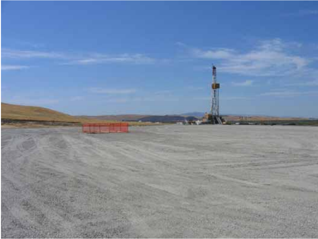
Figure 1 – WS-21 graveled with drilling rig at WS-22 in background, June 20, 2008.
