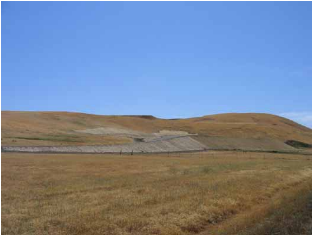
Figure 2 – Jute erosion control blankets installed around WS-23, June 20, 2008.
