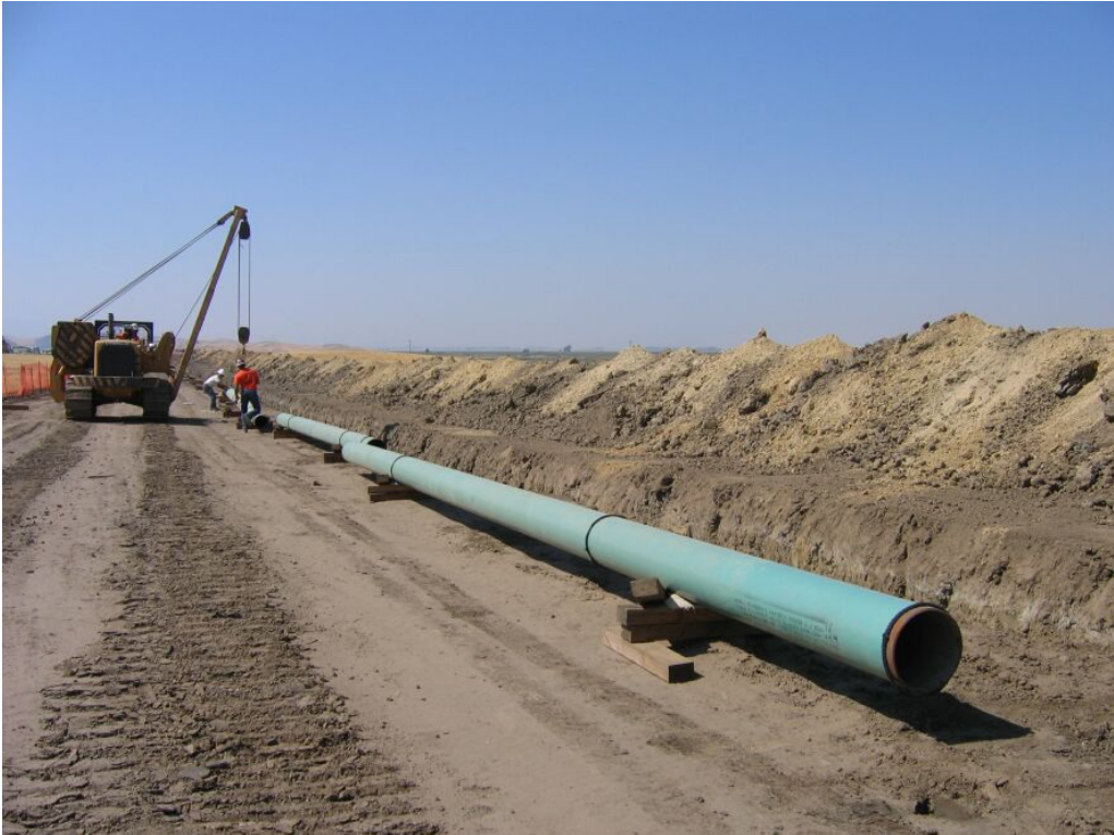
Figure 2 – Pipe stringing along pipeline between Compressor Station and WS-21, July 24, 2008.
