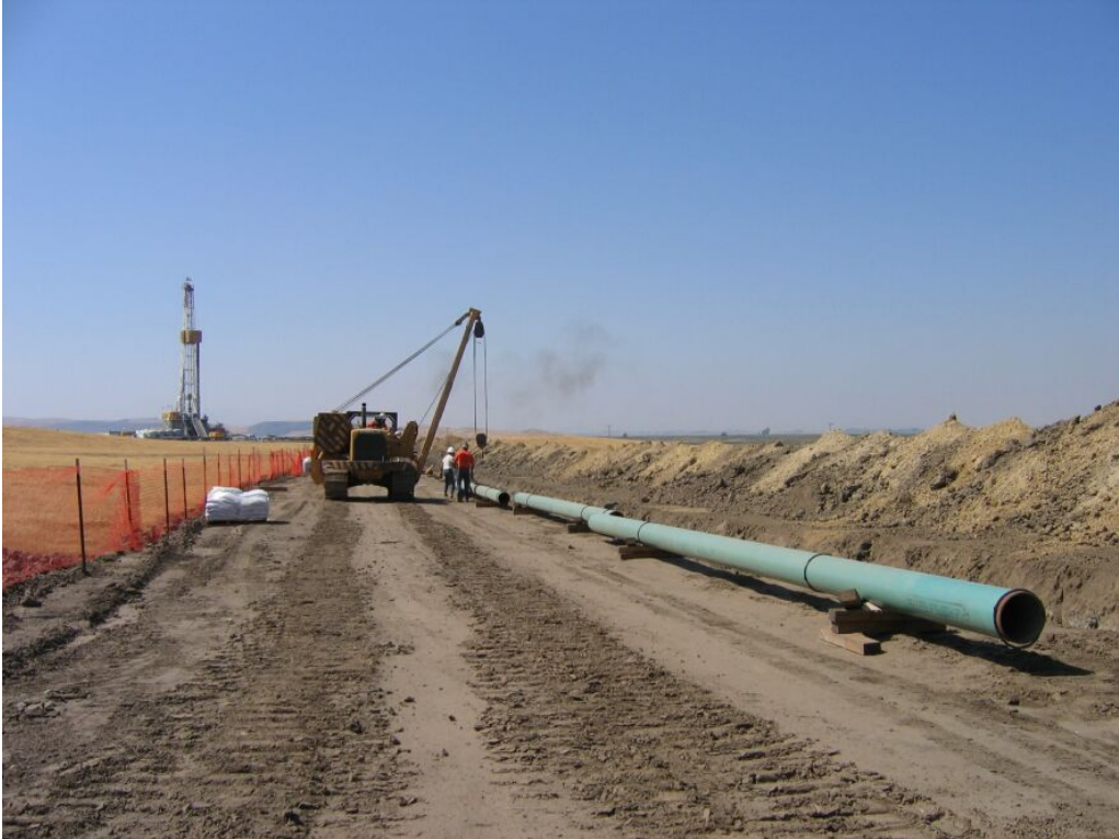
Figure 1 – Drilling rig drilling at WS-21-5 at well pad WS-21 (background) and pipe stringing along pipeline between Compressor Station and WS-21, July 24, 2008.
