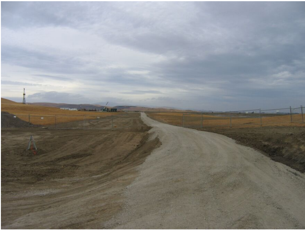
Figure 3 – Right-of-way between the compressor station and WS-21, October 3, 2008.
