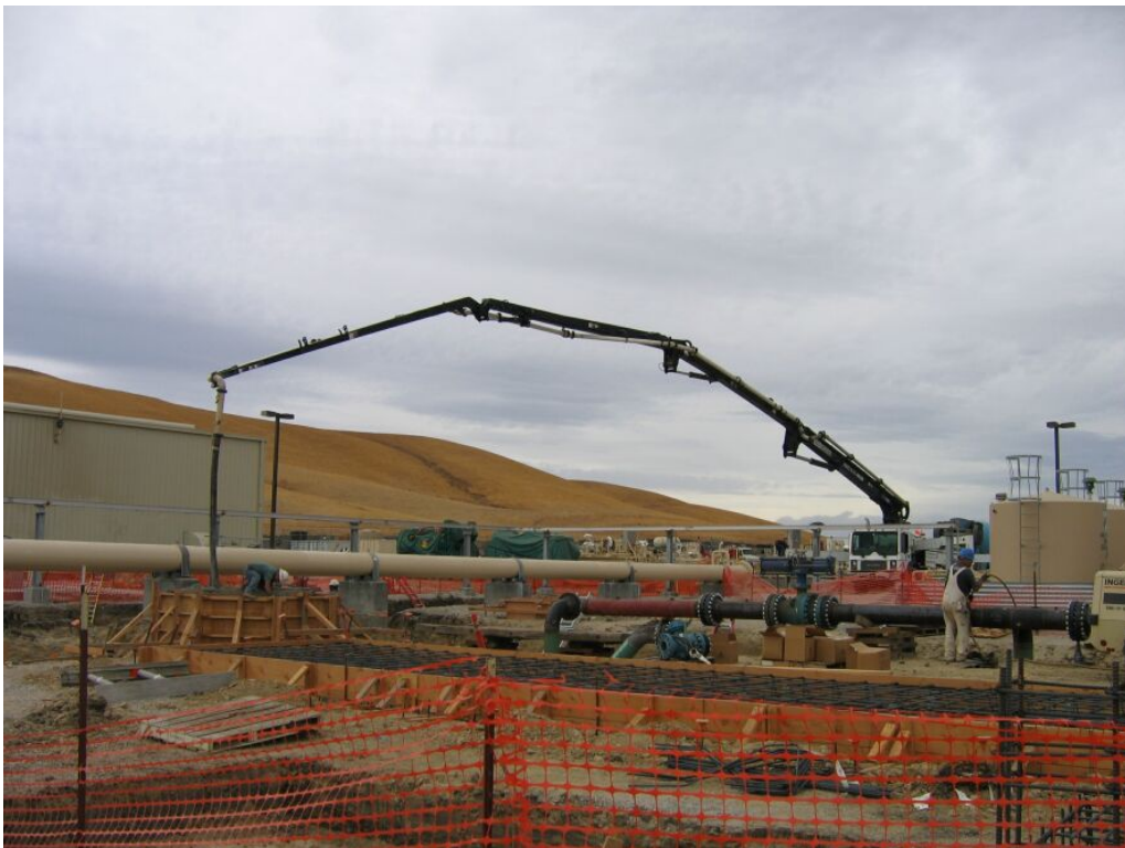
Figure 4 – Pouring cement foundations at the Compressor Station, October 3, 2008.
