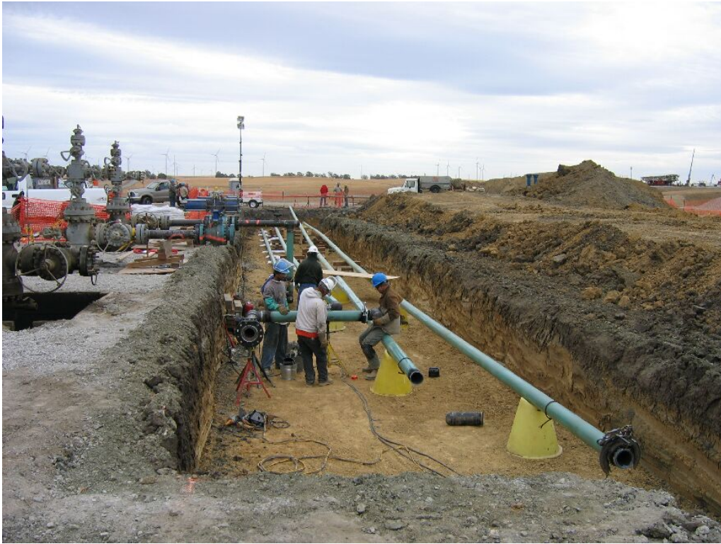
Figure 1 – Crews working on piping at WS-22, October 3, 2008.
