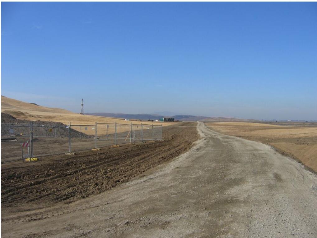
Figure 4 – Pipeline right-of-way from Compressor Station to well sites, October 29, 2008.
