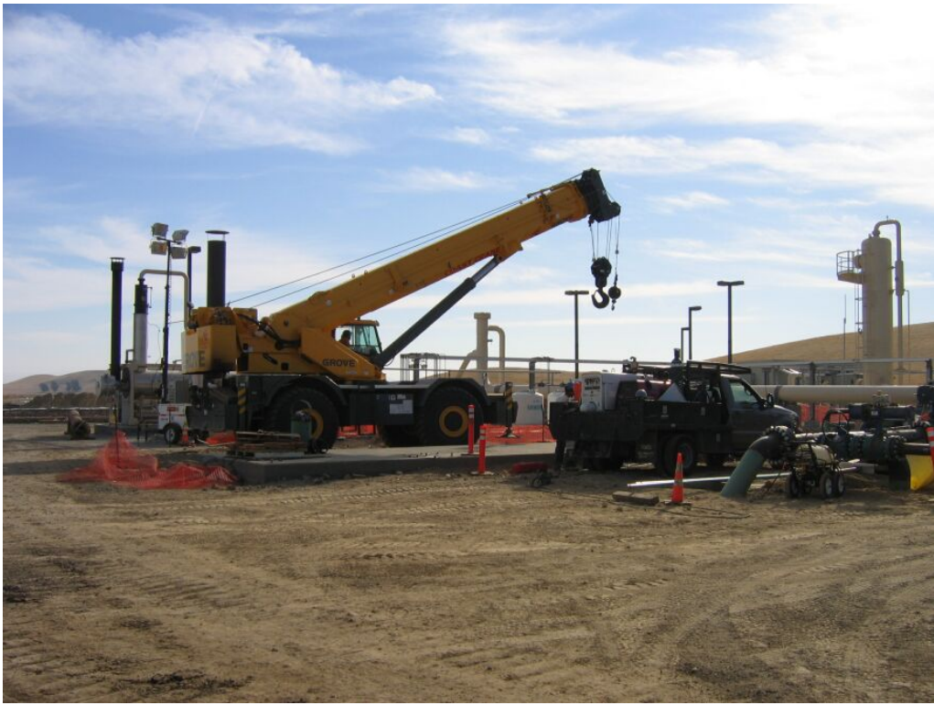
Figure 5 – Crews working at Compressor Station, October 29, 2008.
