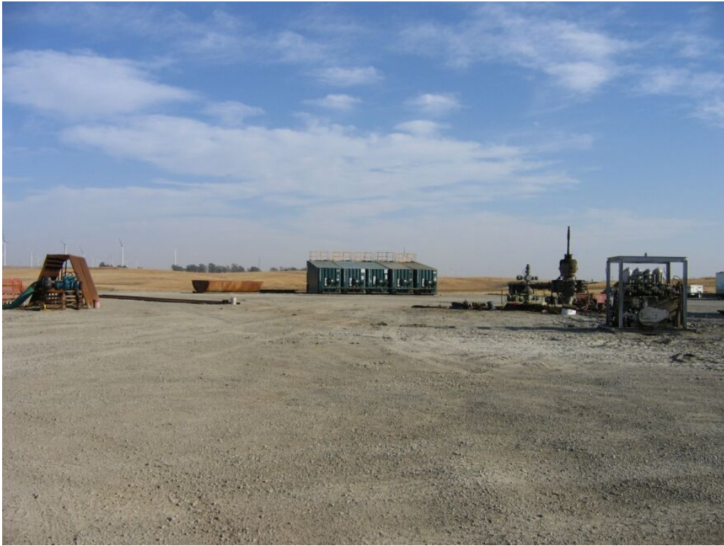
Figure 1 – Well site 21 (WS-21), October 17, 2008.
