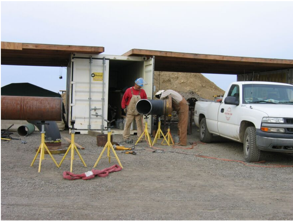
Figure 5 – Crews welding and conducting pipe fabrication at the compressor station, December 12, 2008
