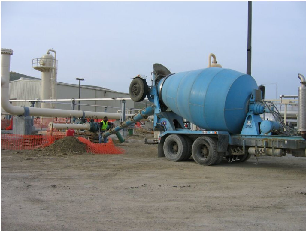
Figure 4 – Crews pouring cement for foundations at the compressor station, December 12, 2008.
