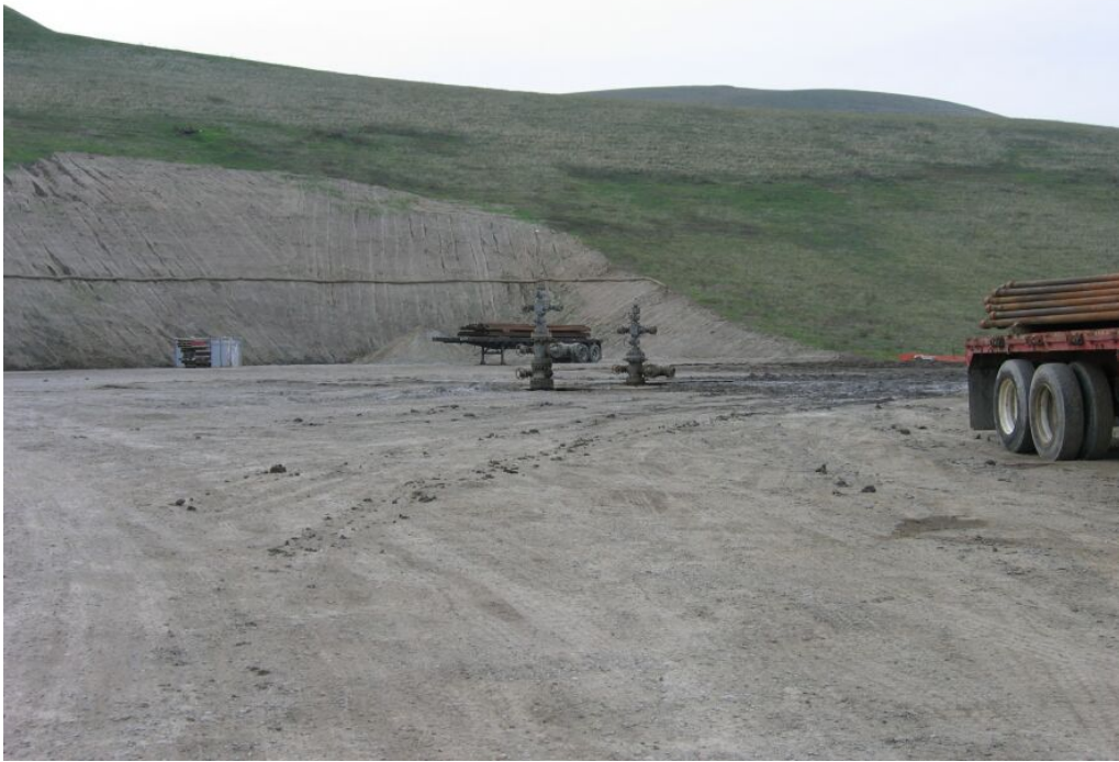
Figure 1 – Workover rig demobilized from well site 23 (WS-23), December 12, 2008.
