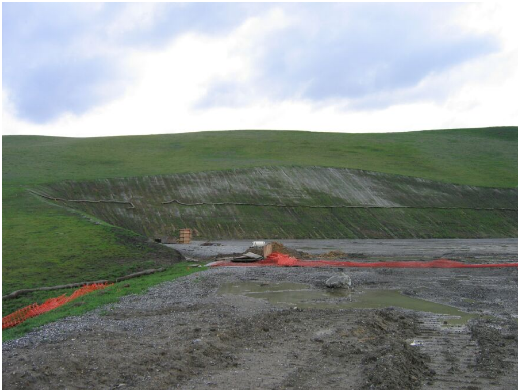
Figure 2 – Cut slope at well site 23 (WS-23) revegetating, February 18, 2009.
