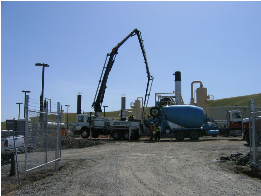
Figure 3 – Crews pouring cement at Compressor Station, May 14, 2009.
