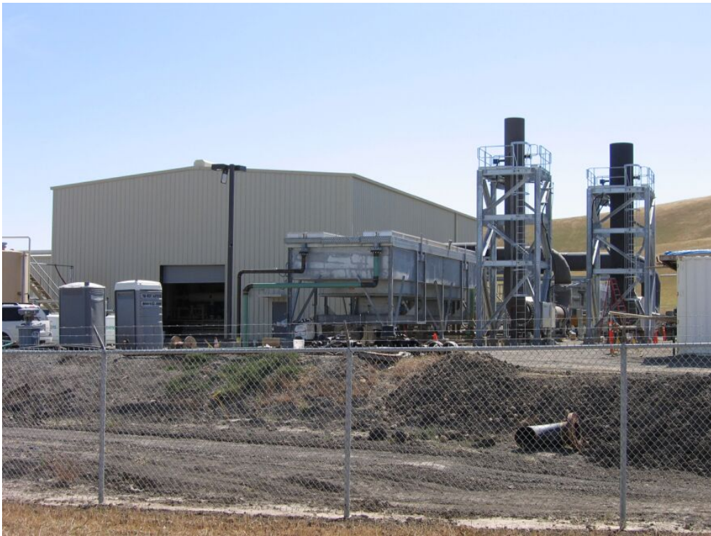
Figure 3 – New compressor building and attached equipment at Compressor Station, May 21, 2009.
