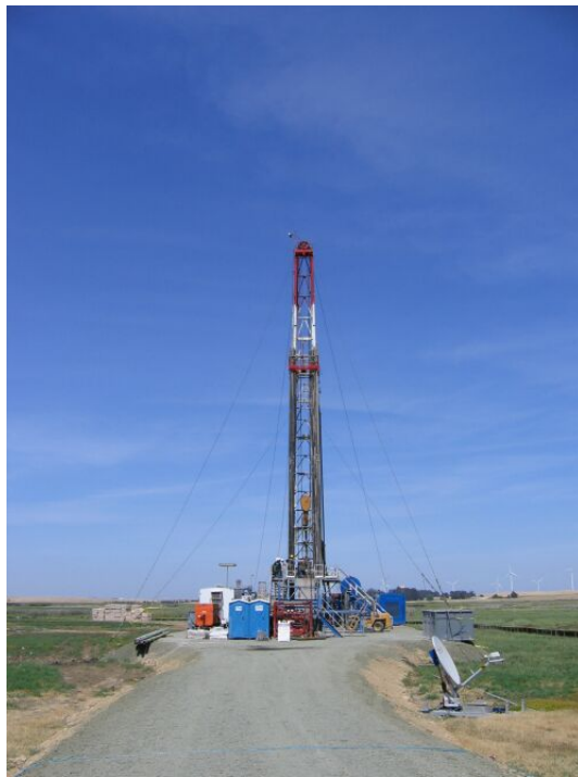
Figure 2 – Drilling rig at Wagenet 5 (W5), May 21, 2009.
