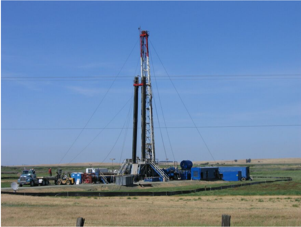
Figure 1 – Drilling at Wagenet 5 (W5), May 21, 2009
