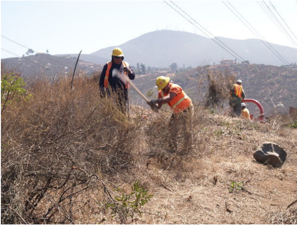
Figure 3 – Crew using hand tools to clear brush. In background, dry brush being reduced with a small chipper.
