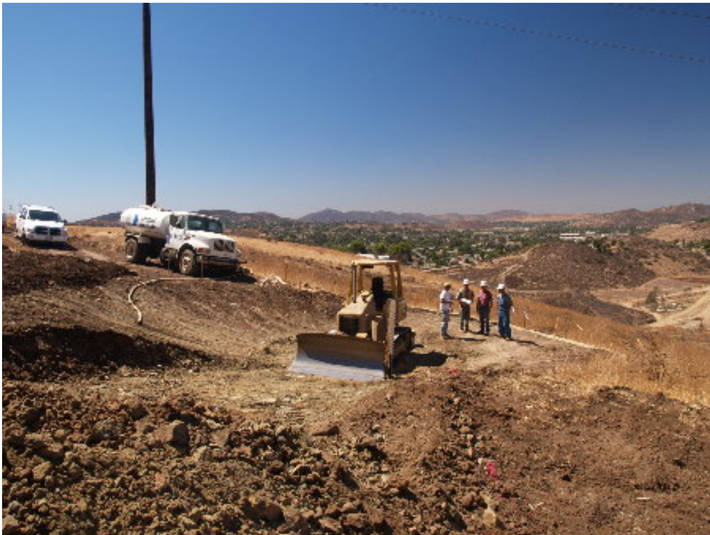
Figure 2 – The grading crew returned to Tower Site 1150 to reconfigure the site.
