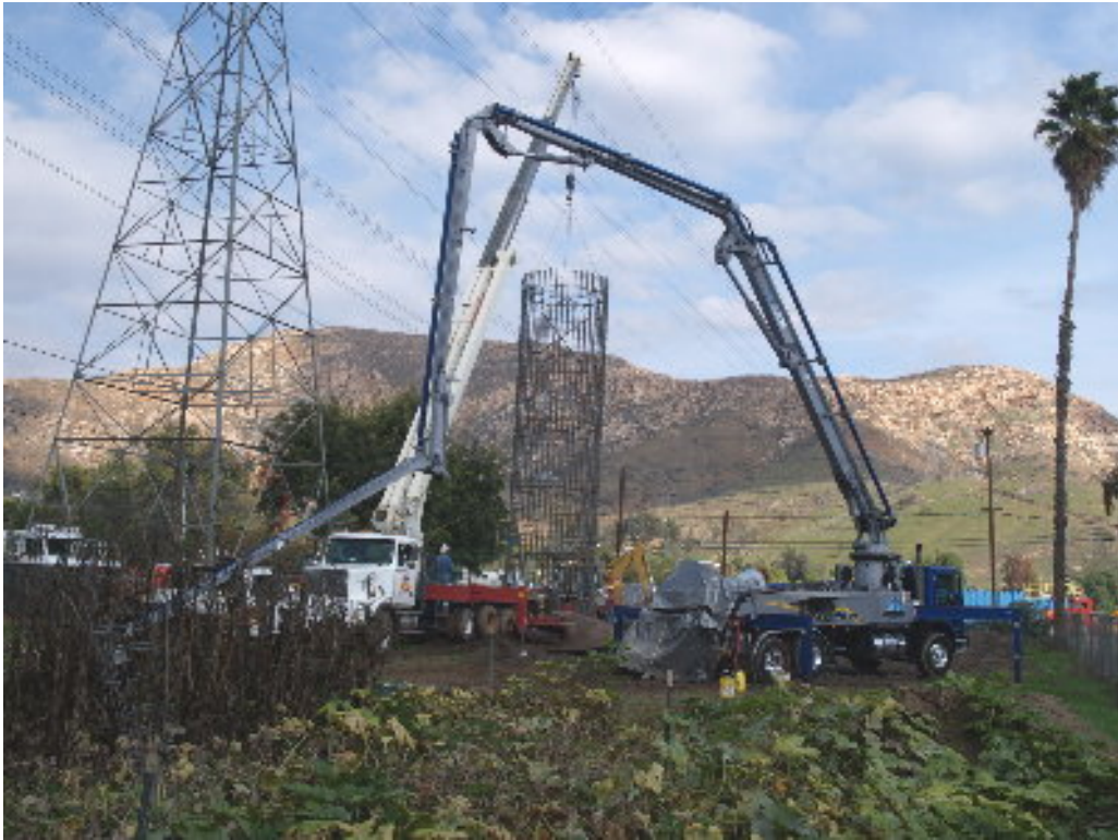
Figure 3 – The concrete pumping truck set up at Tower Site 1210.
