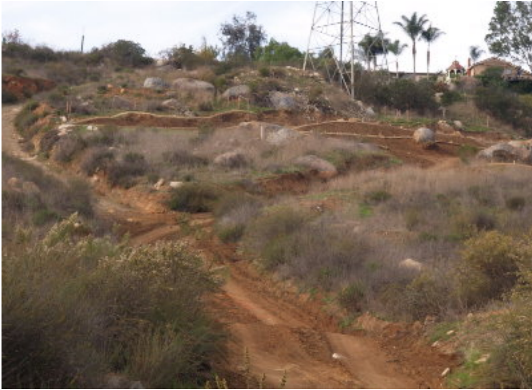
Figure 7 – The BMPs at Tower Site 440 have been repaired.
