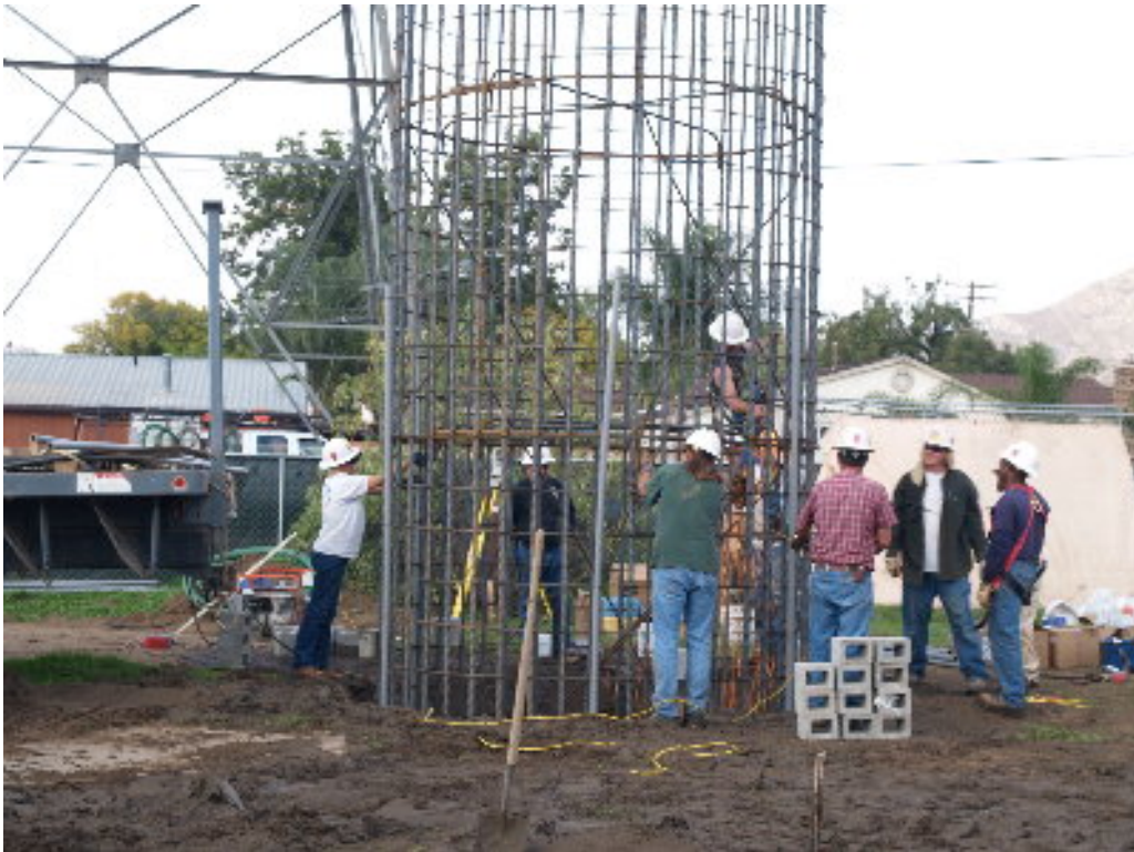
Figure 2 – The crew at Site 1210 worked on the rebar cage.
