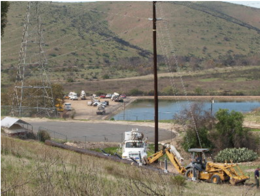
Figure 2 – A PAR crew excavated for support anchors east of Santee Lakes.
