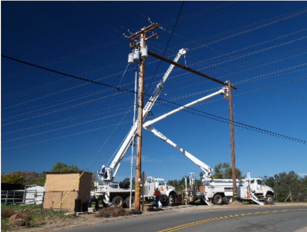
Figure 3 – The PAR transmission crew raised braces for the stringing operation.
