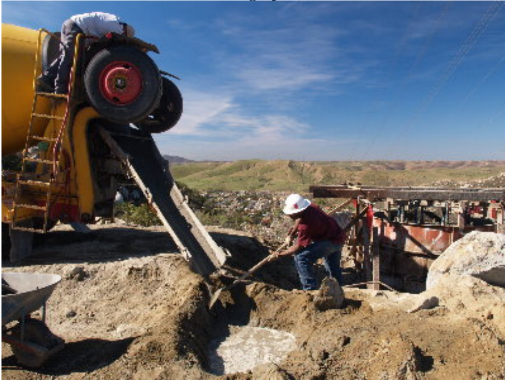
Figure 1 – The concrete truck at Tower Site 1300 was properly washed-out on-site.
