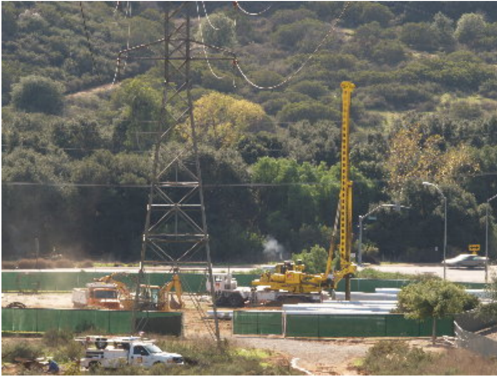
Figure 5 – The drill worked on foundations at Steele Canyon High School.
