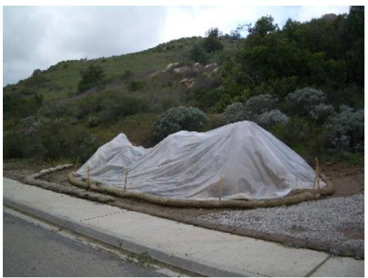
**Figure 2** – Spoil piles were covered to prevent erosion during the recent rains. The straw waddles installed are not sufficient to contain the material in the pile.
