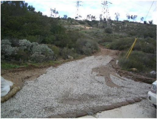
Figure 3 – Sandbags and rock were used to prevent sediment transport onto public roads.
