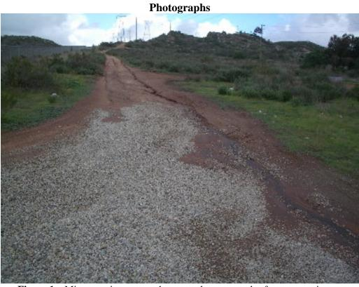
Figure 1 – Minor erosion occurred at several access roads after recent rains. No environmental impacts were noted.
