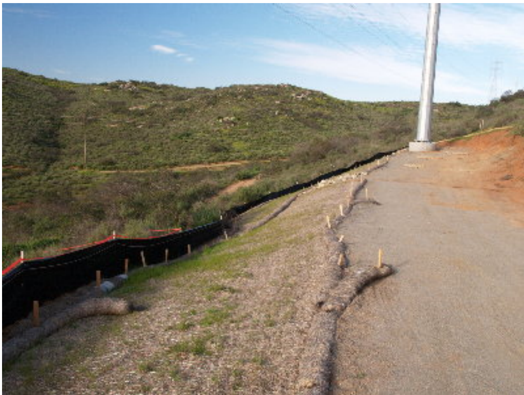
Figure 4 – SDG&E has made improvements to the BMPs at Pole Site 321.
