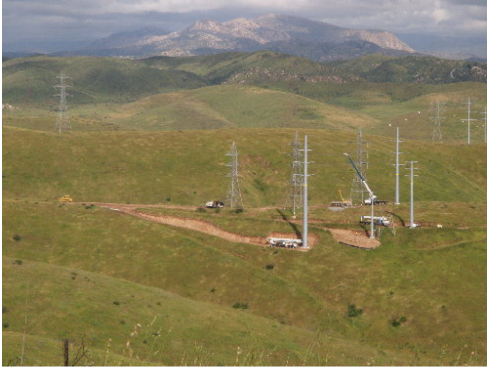
Figure 1 – An SDG&E transmission line crew worked at Fanita Junction moving lines.
