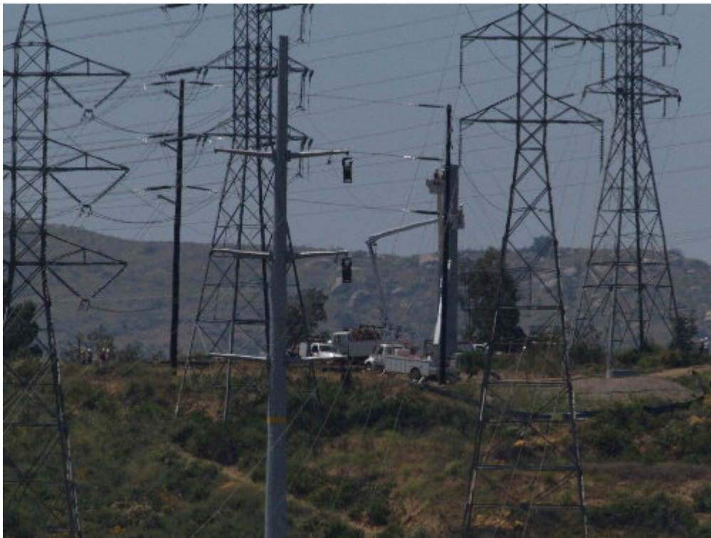
Figure 2 – The Wilson stringing crew pulling line across Lake Jennings Road.
