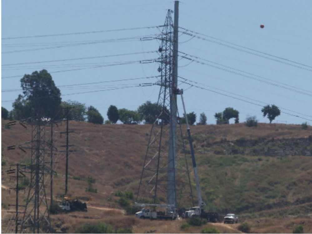
Figure 1 – Wilson crews prepared for the line pull across Lake Jennings Road.
