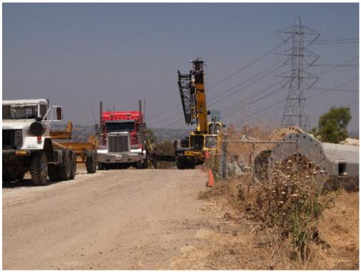
**Figure 3** – Steel pole sections were delivered to the Miguel Substation staging area for the next phase of construction.
