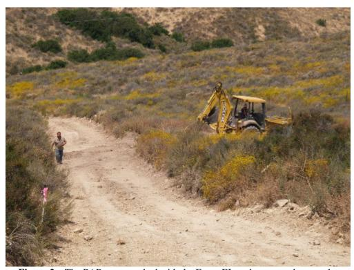
**Figure 2** – The PAR crew worked with the Essex EI to place water bars on the access road down from Pole Site 10. The backhoe is operating on an access road, not in native vegetation.
