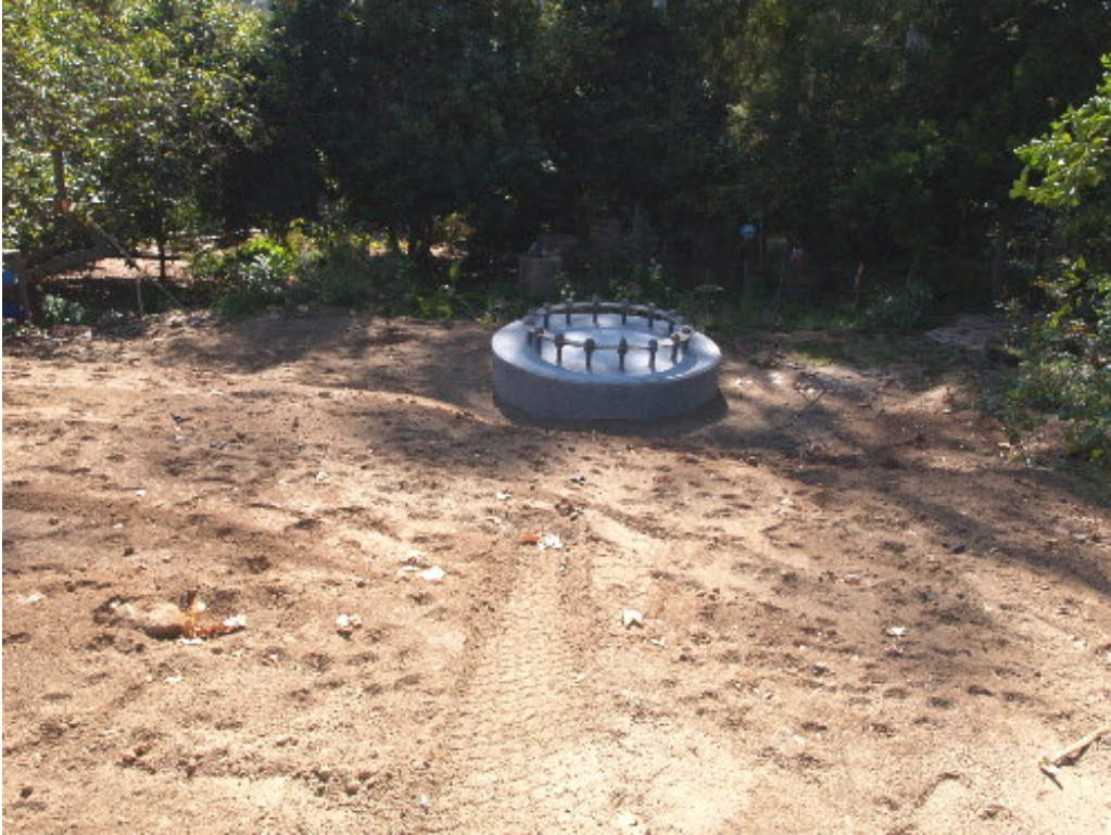
Figure 1 – The Tri-State drilling crew completed the foundation at Vista Rodeo.
