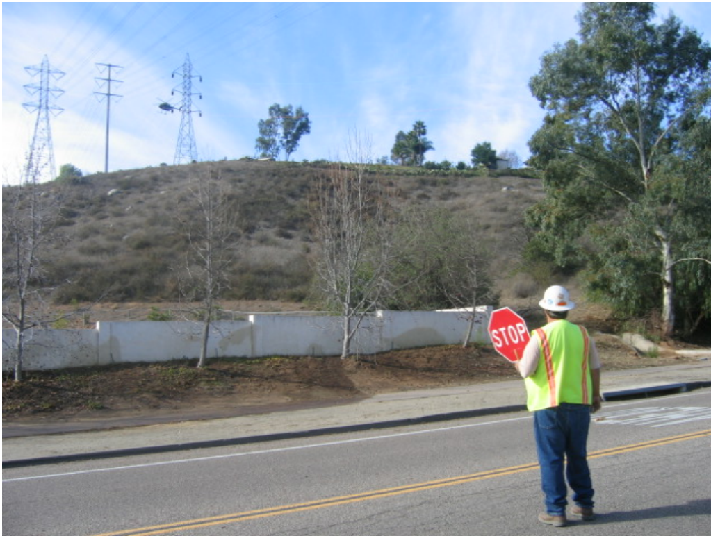
Figure 3 – Traffic control was in place during rope installation across Hillsdale Road.
