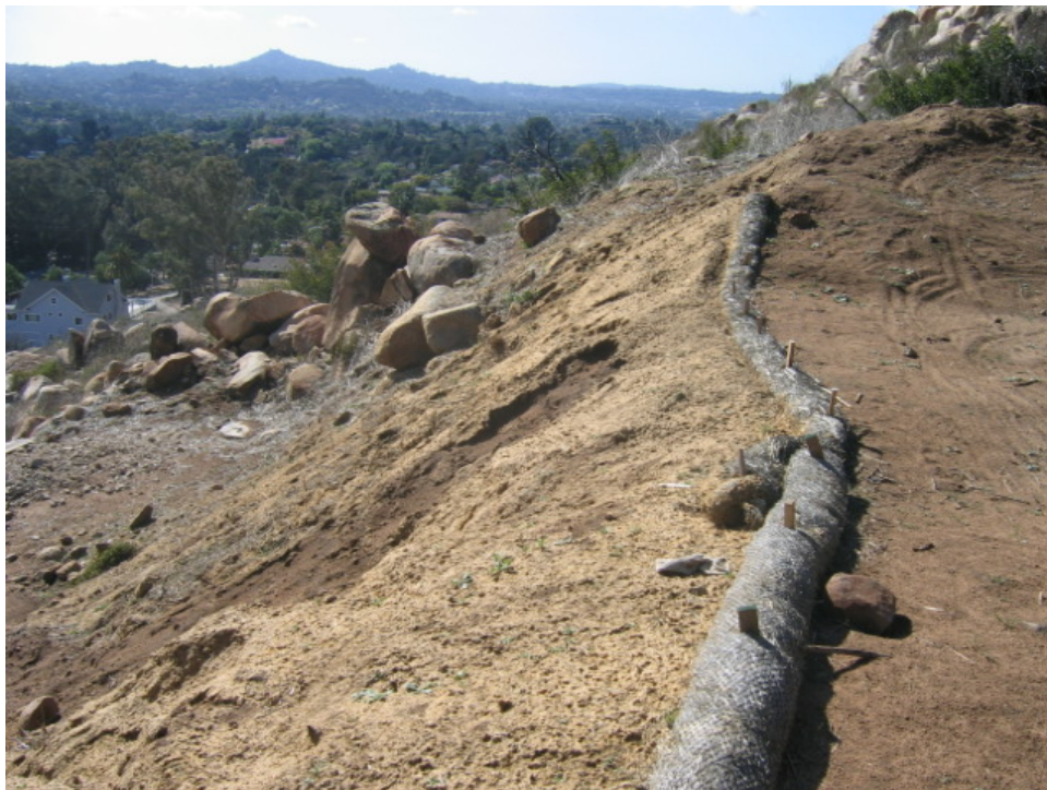
Figure 2 – Hydro-seeded area off Camino Monte Sombre. After recent rain events, some of the hydro-seeded slope has sloughed off.
