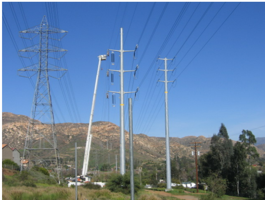
Figure 2 – Par crews clipping in wire near Highway 67.
