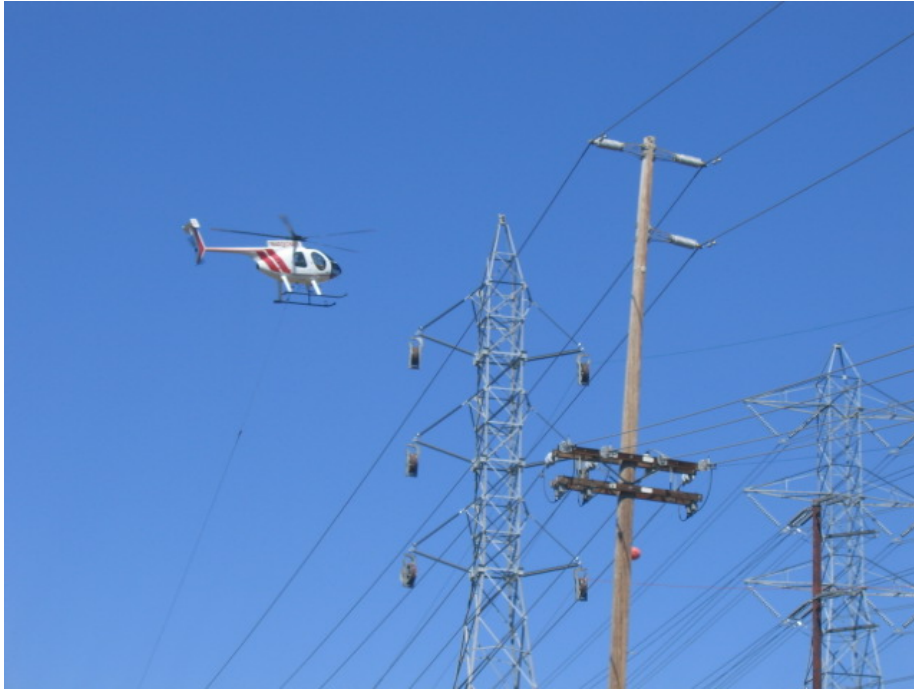
Figure 1 – Skyline installation along Lake Jennings Road.
