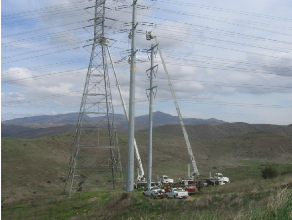
Figure 1 – Par crews dead-ending wire near Santee Lakes.
