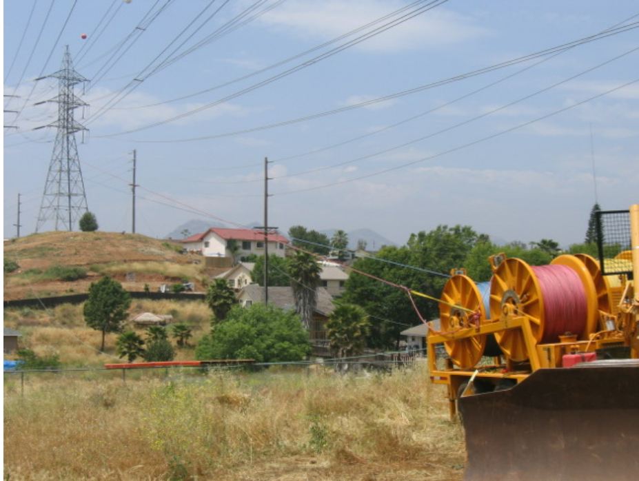
Figure 1 – Sturgeon crews working on the temporary 230 kV lines near Lake Jennings. The “put back” involves reconfiguring the wood poles to accommodate a double circuit of smaller kV lines.
