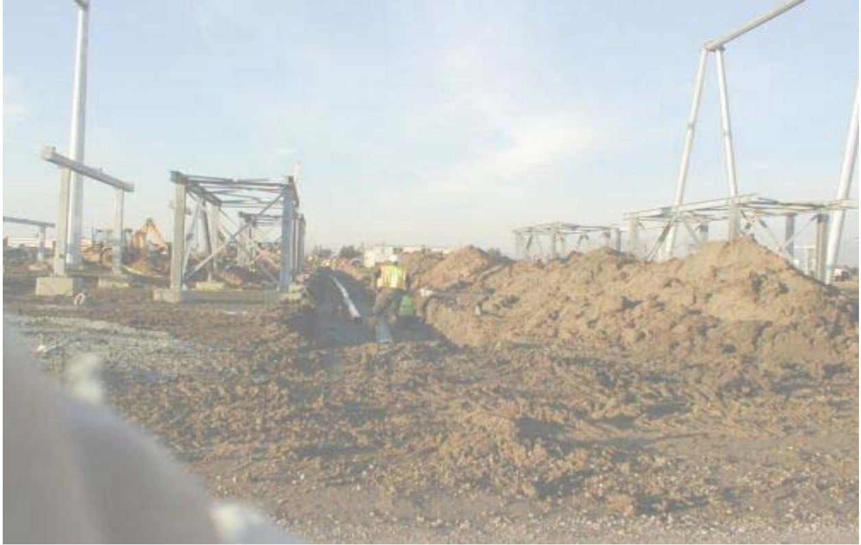
Figure 4 Underground Pipe Installation at the Los Esteros Substation January 3, 2003
